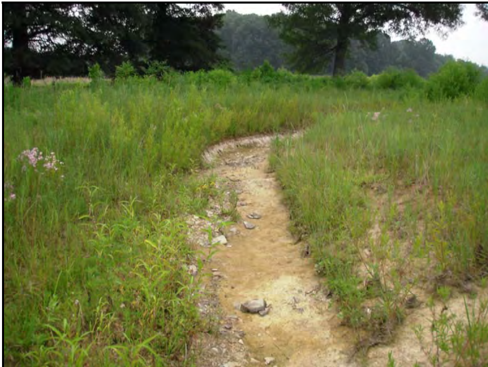
Stream Photo # 6 Constructed Riffle Looking Downstream at Sta. 136+00
