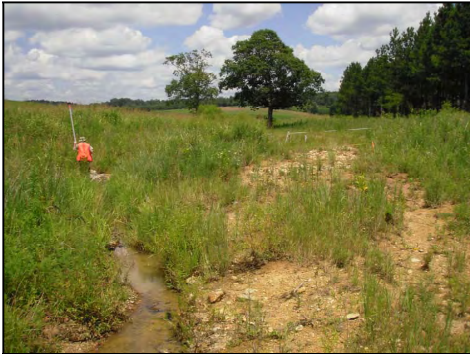
SPA # 4. Right bank erosion at Sta. 437+00.
