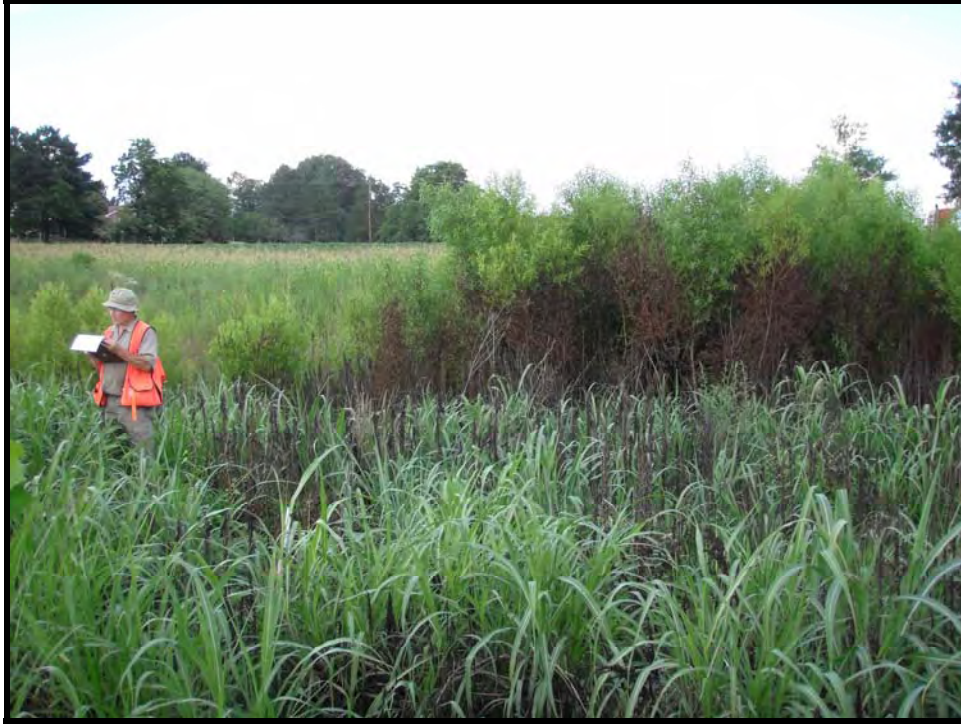
VPA1. Dead vegetation along channel. Sta. 107+50
