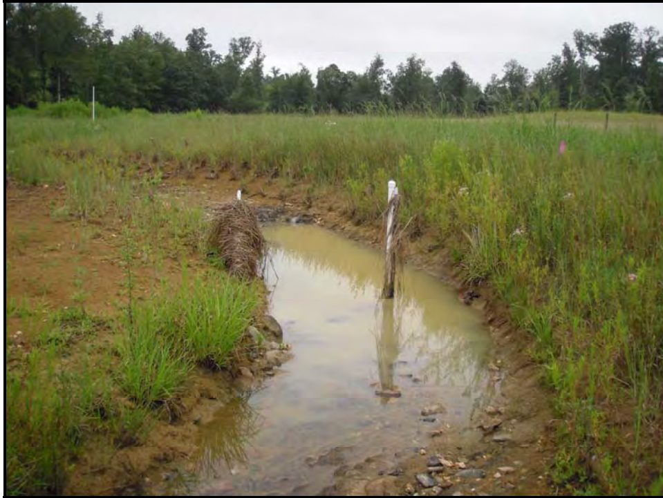
Stream Photo # 9 Rack lines at Crest Gauge 3 at Sta. 164+25
