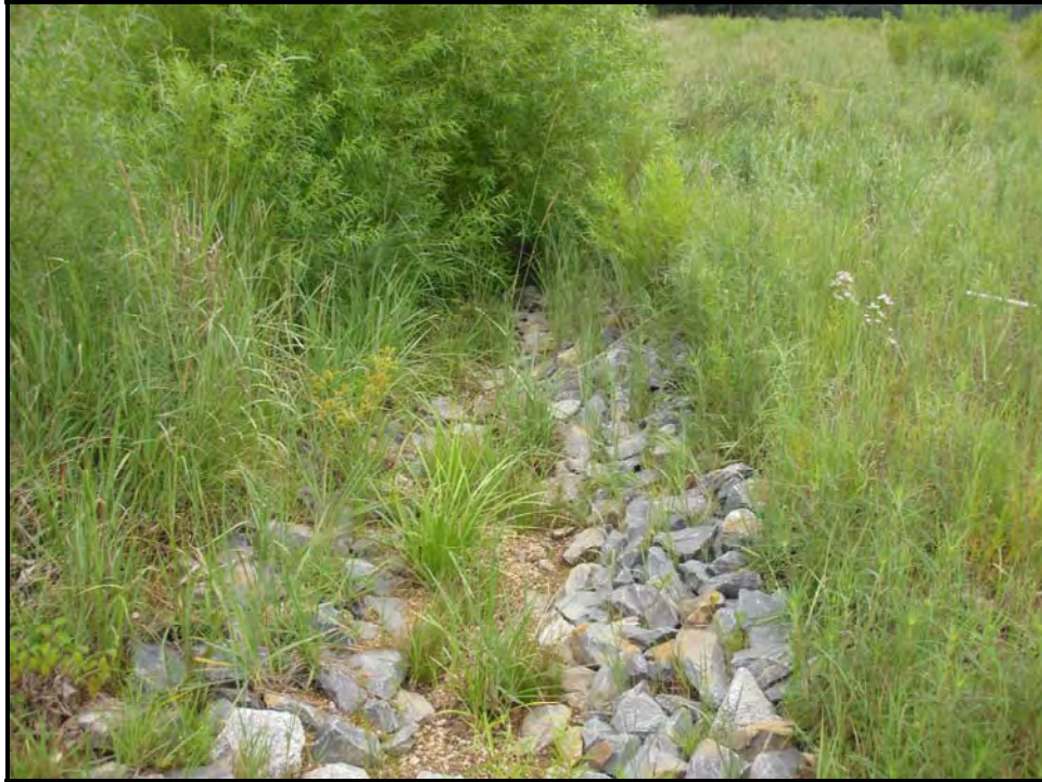
Stream Photo # 13 Constructed Riffle Looking Downstream at Sta.302+10
