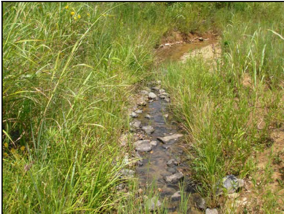
Stream Photo # 24 Constructed Riffle Looking Downstream at Sta. 443+45
