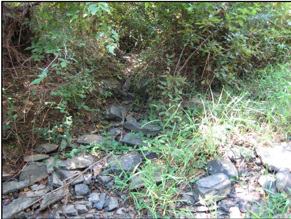
Stream Photo # 10 Upstream end of UT-2 at Sta. 179+00
