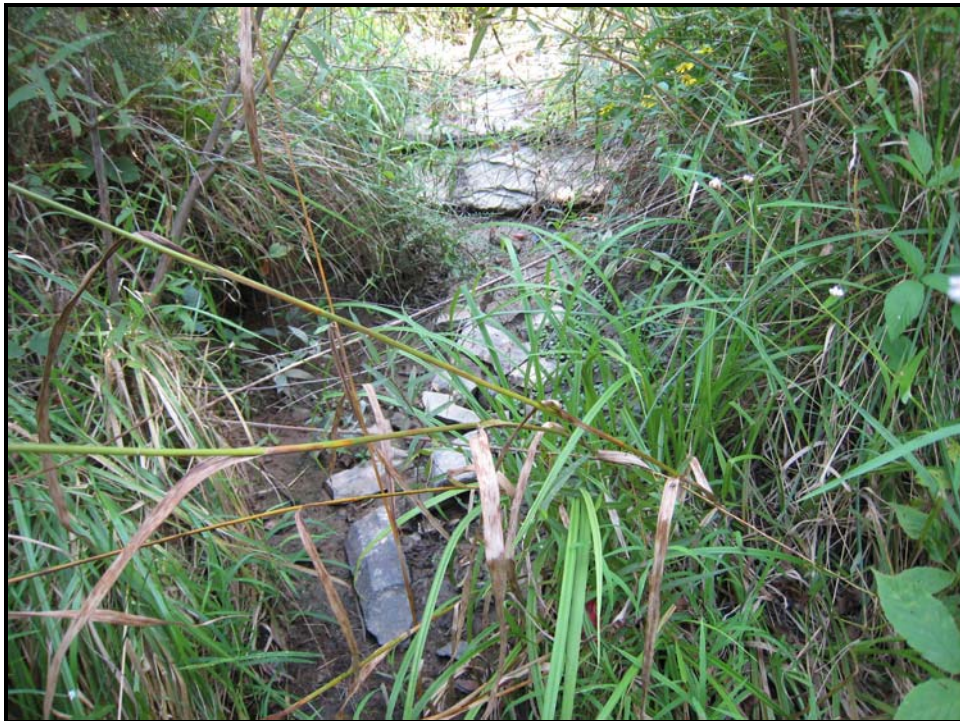
Stream Photo # 12 Rock Cross Vane Looking Upstream at Sta. 206+00
