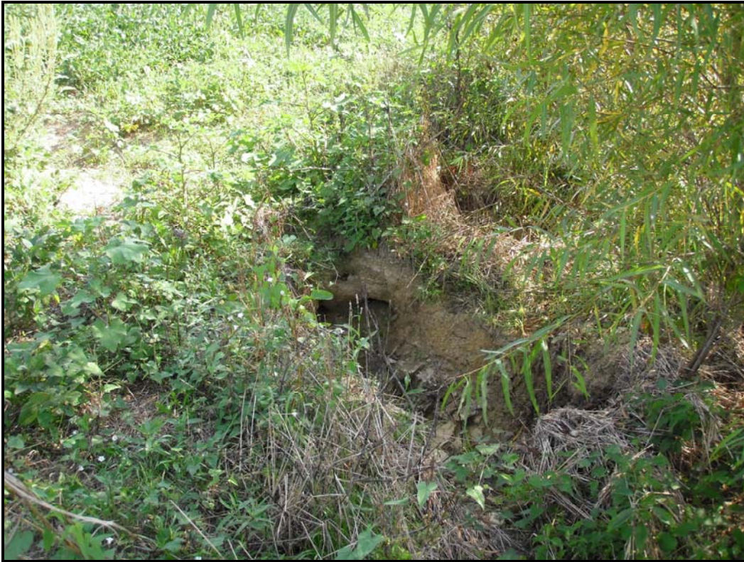
VPA4. Minor erosion forming a headcut at cultivated field edge and buffer.
