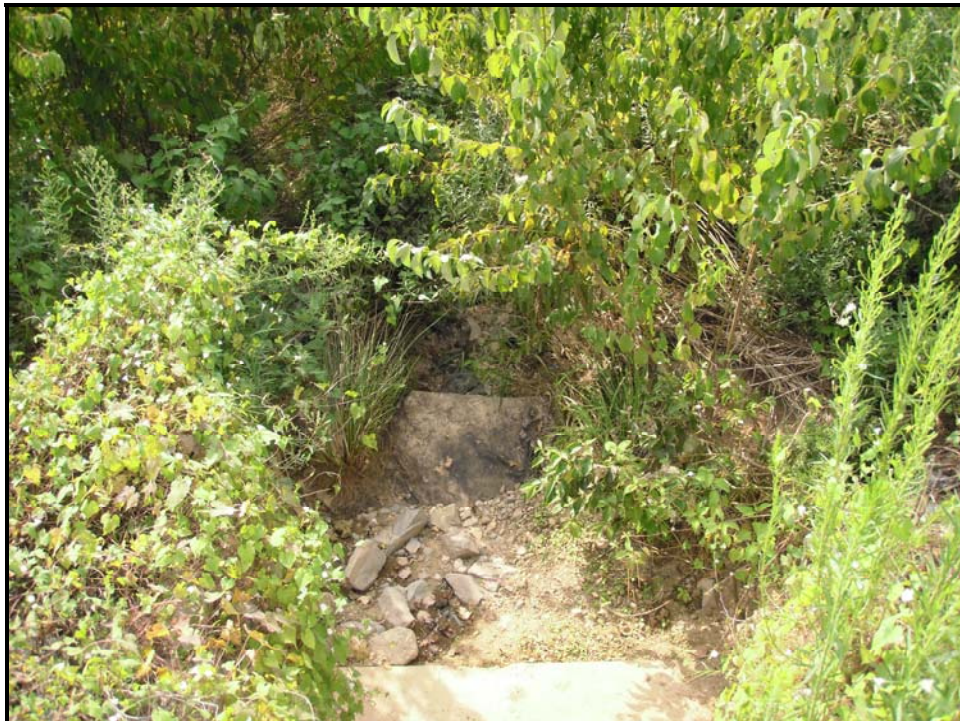
Stream Photo # 2 Rock Cross Vane Looking Downstream at Sta. 116+75
