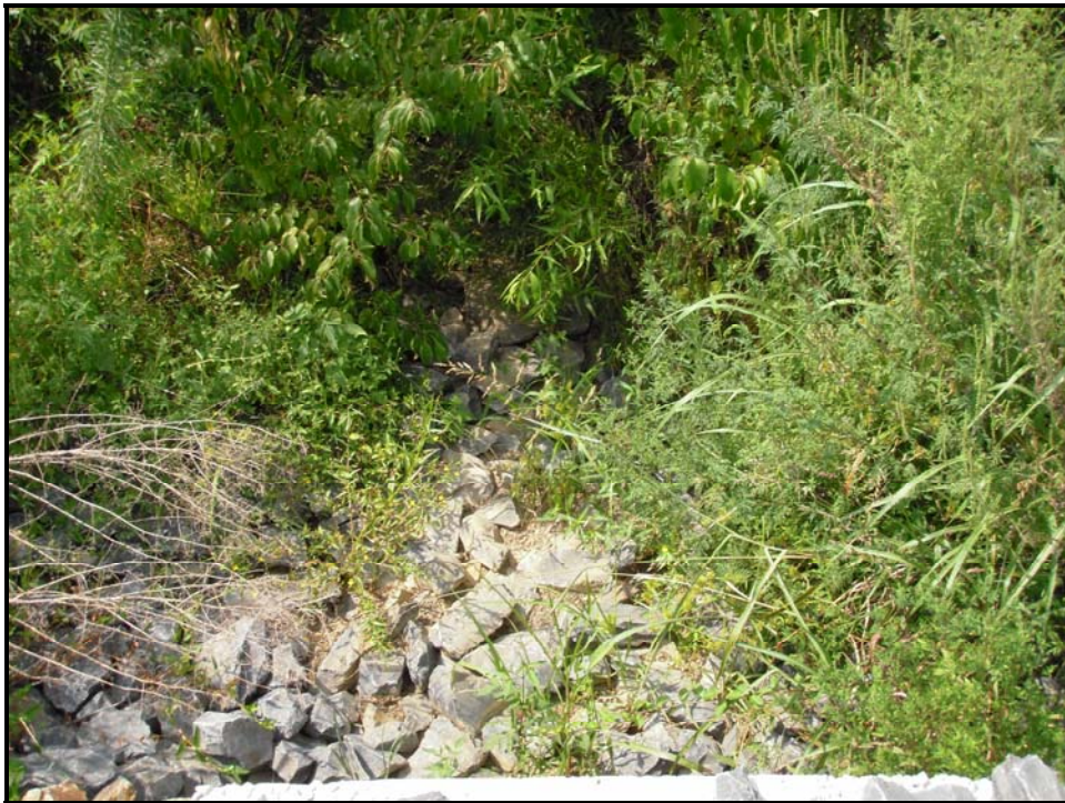
Stream Photo # 18 Downstream at Sta. 416+35
