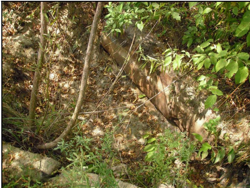
Stream Photo # 6 Rock Cross Vane Looking Downstream at Sta. 141+77
