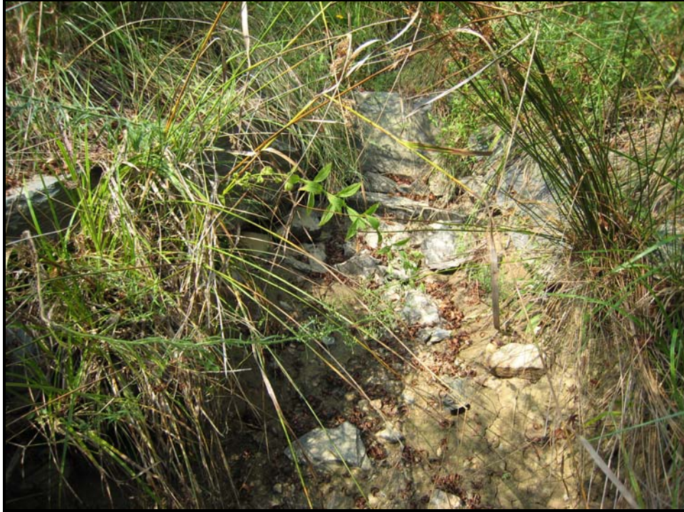
Stream Photo # 15 Rock Cross Vane Looking Upstream at Sta. 308+30
