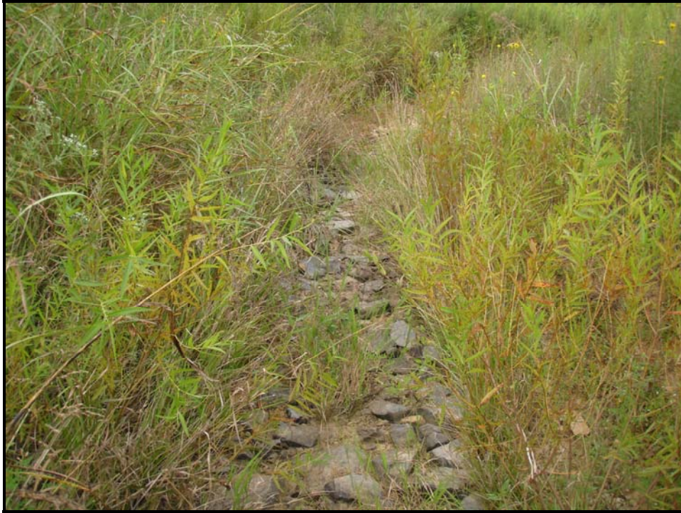
Stream Photo # 23 Constructed Riffle Looking Downstream at Sta. 443+45
