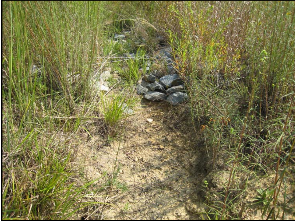
Stream Photo # 13 Constructed Riffle Looking Downstream at Sta.302+90
