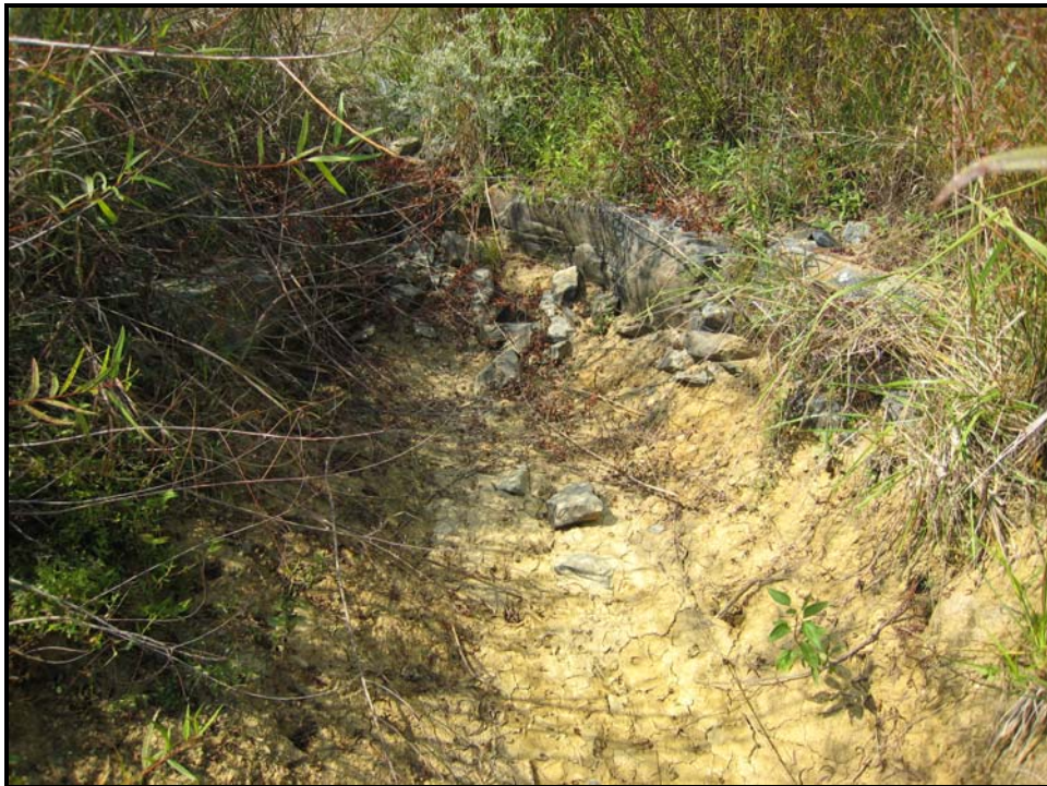
Stream Photo # 14 Rock Cross Vane Looking Upstream at Sta. 304+74
