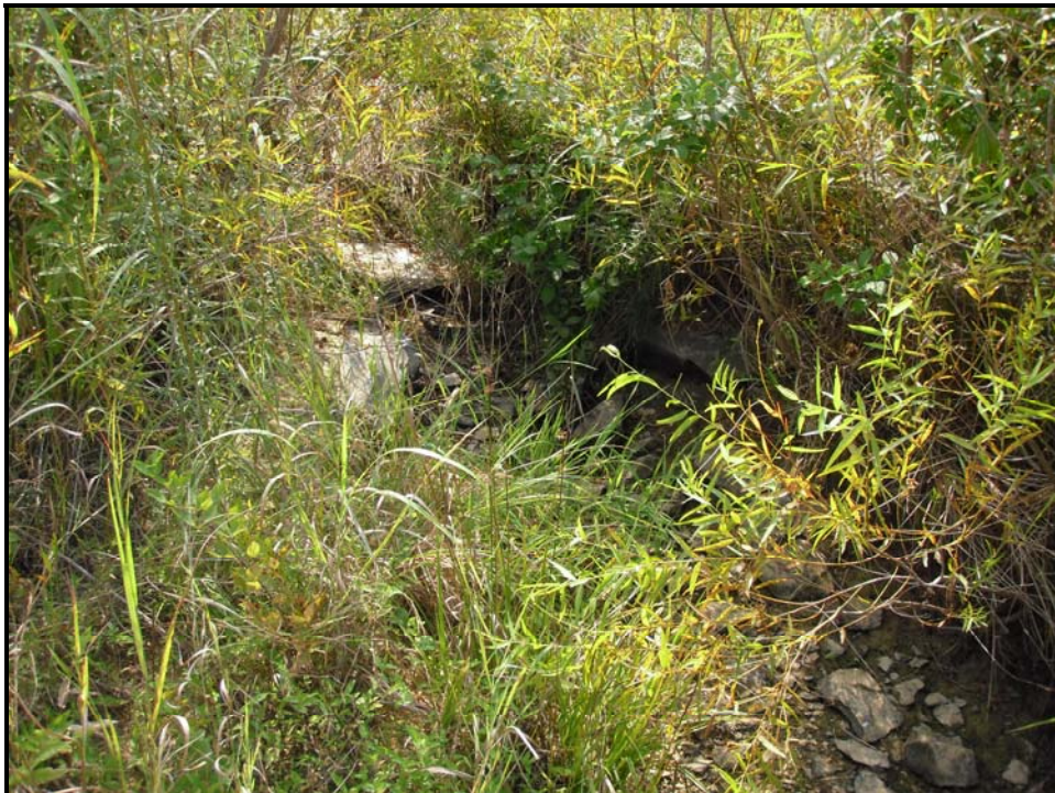
Stream Photo # 20 Rock Cross Vane Looking Upstream at Sta. 436+00
