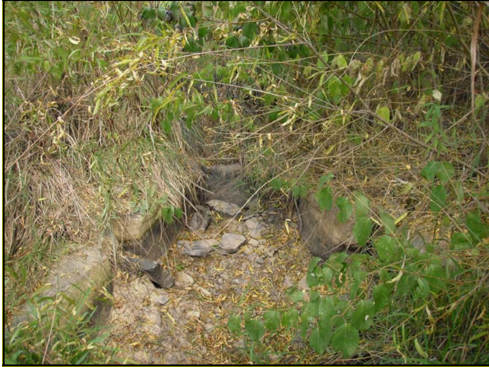
Stream Photo # 3 Rock Cross Vane Looking Upstream at Sta. 118+15
