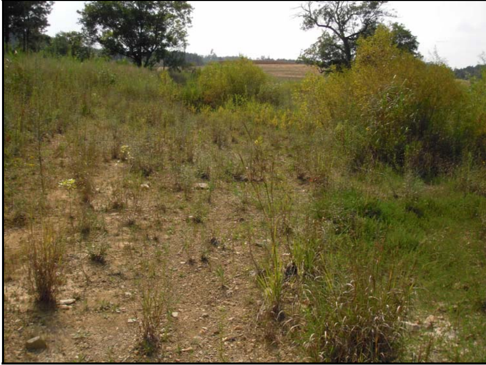
SPA #5. Right bank erosion at Sta. 437+00.
