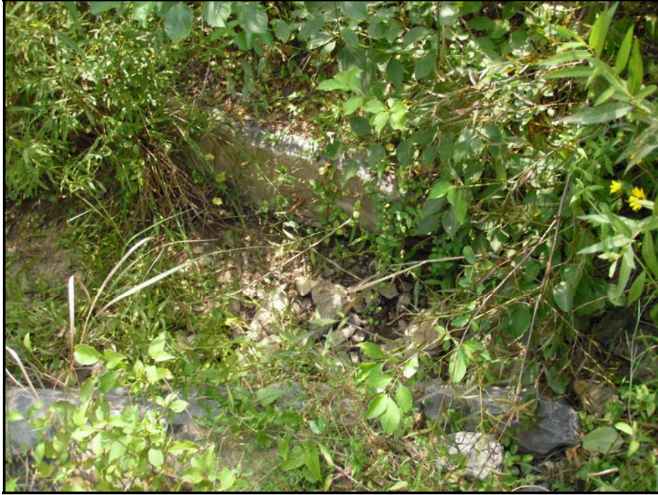
Stream Photo # 17 Rock Cross Vane Looking Downstream at Sta. 413+50
