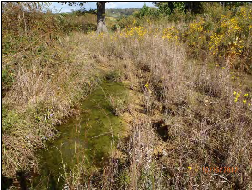
SPA # 4. Right bank erosion at Sta. 437+00.
