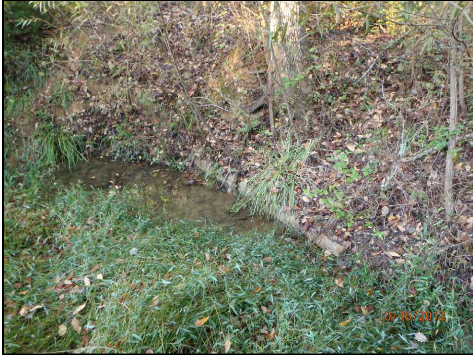
Stream Photo # 17 Log Cross Vane Looking Downstream at Sta. 410+95
