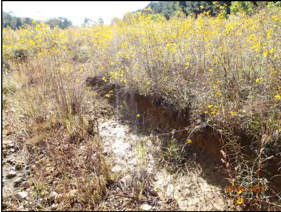
SPA # 1. Minor right bank erosion at Sta. 148+00.
