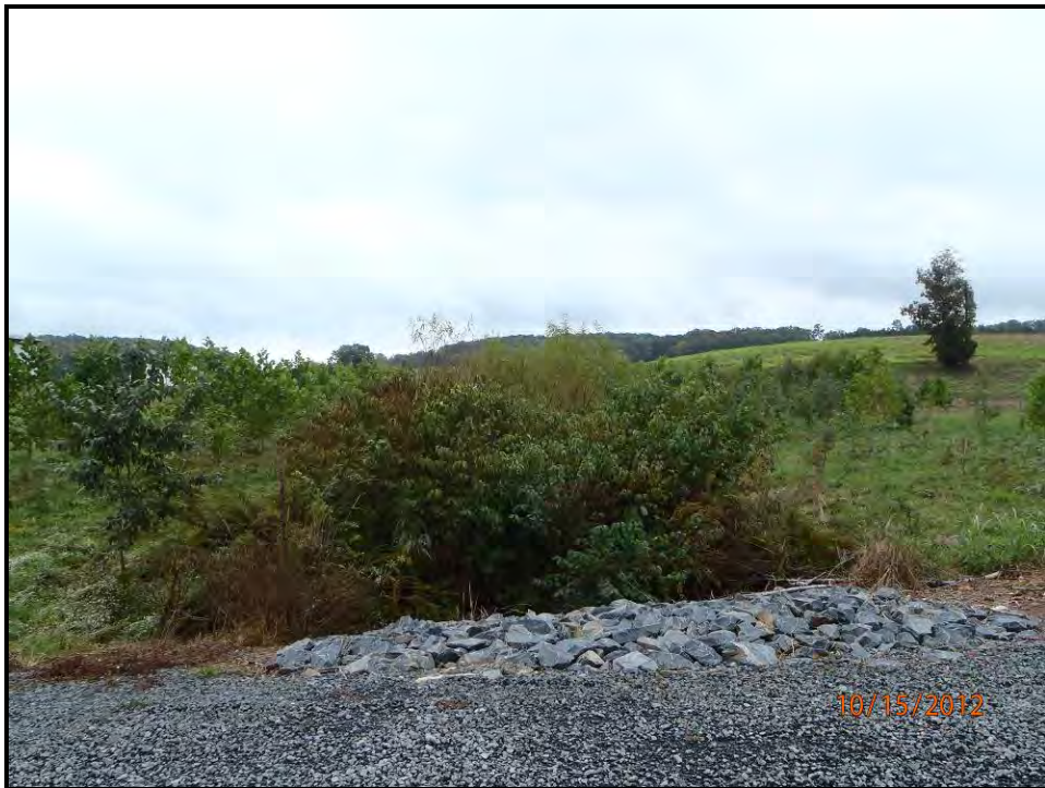
Stream Photo # 2 Looking Downstream from Road Crossing at Sta. 116+75
