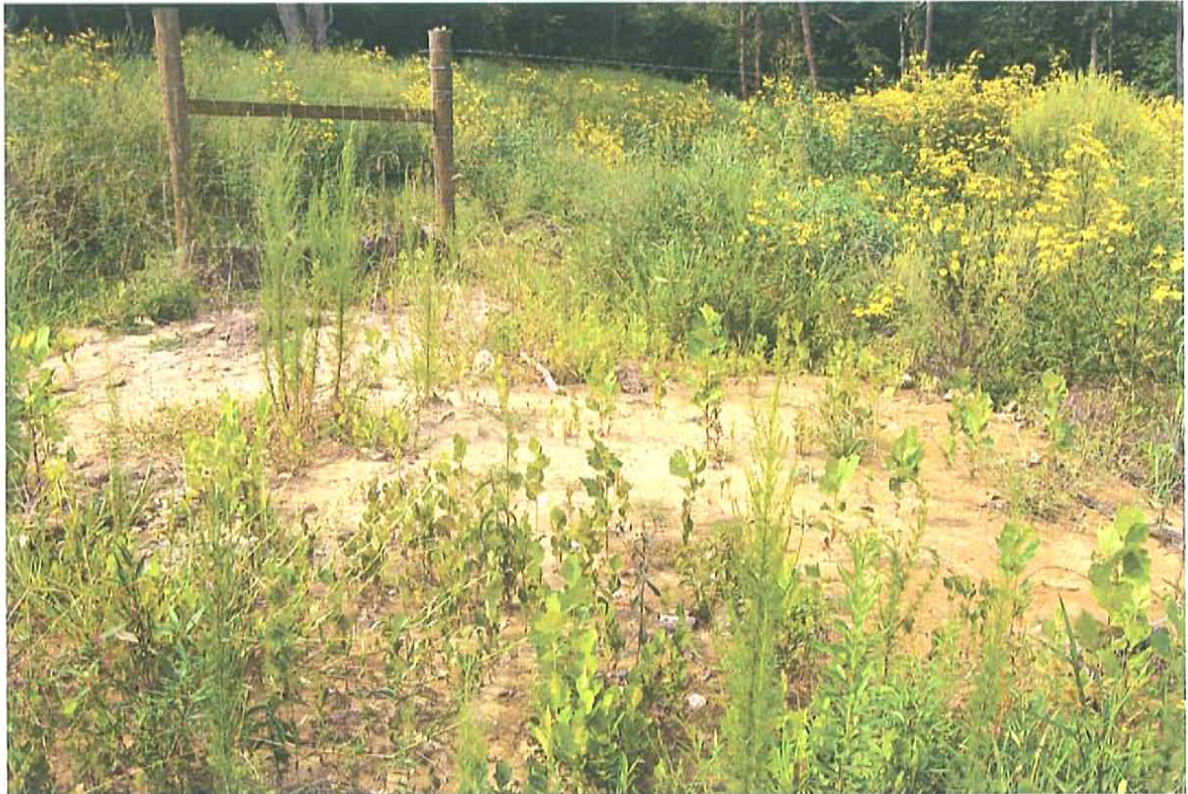
Rocky Branch (Station 1+77) View near I-77 right-of-way fence of eroded area caused by a debris jam. Area is currently vegetated with natural sycamore seedlings.
