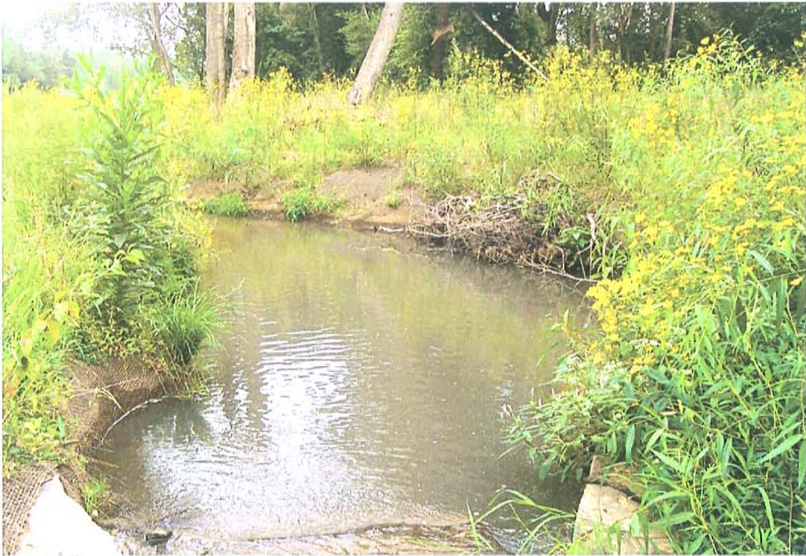
Rocky Branch (Station 22+32) Cross Section 6 – Pool. Large cross sectional area compared with proposed design.
