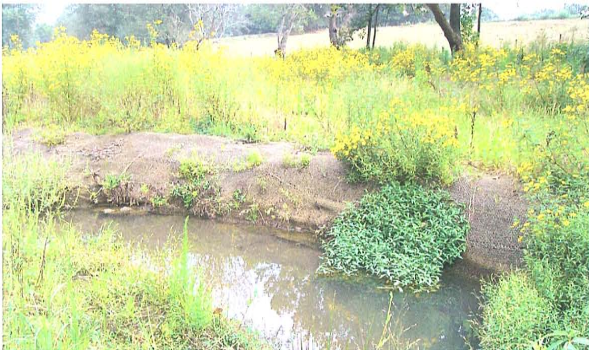
Rocky Branch (Stations 32+80 – 33+00) Area of sloughing banks. View looking across channel from left to right.
