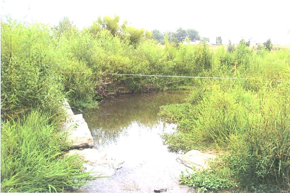
Cross Section 1 - Pool. (Rocky Branch, STA 4 + 25) View looking downstream.
