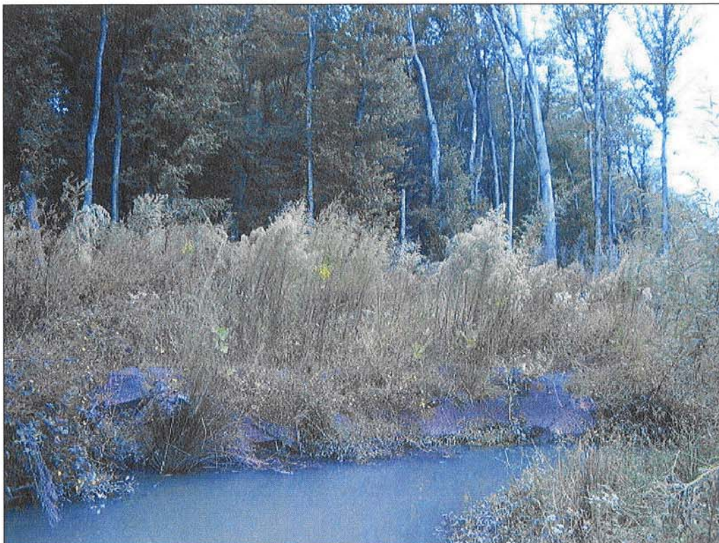
STREAM PROBLEM AREA 3: ROCKY BRANCH (STATIONS 25+70 - 25+80) STRETCH OF CHANNEL WITH SLOUGHED BANKS. VIEW LOOKING ACROSS CHANNEL FROM RIGHT TO LEFT.
