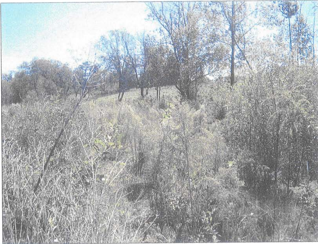
PHOTO POINT 4. VIEW LOOKING EAST TOWARD NEWLY CONSTRUCTED TRIBUTARY I AND MAIN CHANNEL.
