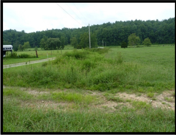
UT 2 looking downstream, across culvert, at straightened channel.
