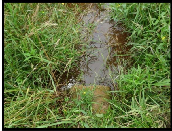
Culvert on UT 2.
