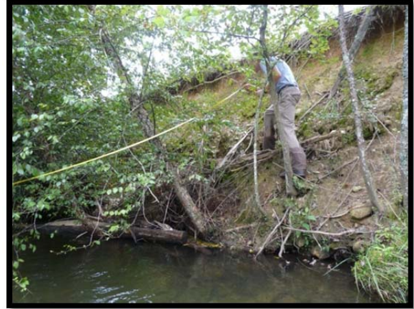
Looking slightly upstream at left vertical bank of Roses Creek
