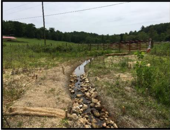
3.19 Conveyance created at STA 20+75 (Roses Creek)
