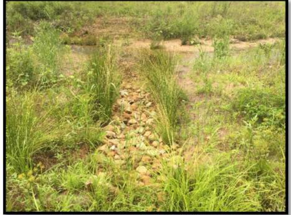
3.22 Repaired hole converted to a floodplain interceptor STA 38+69 (Roses Creek)
