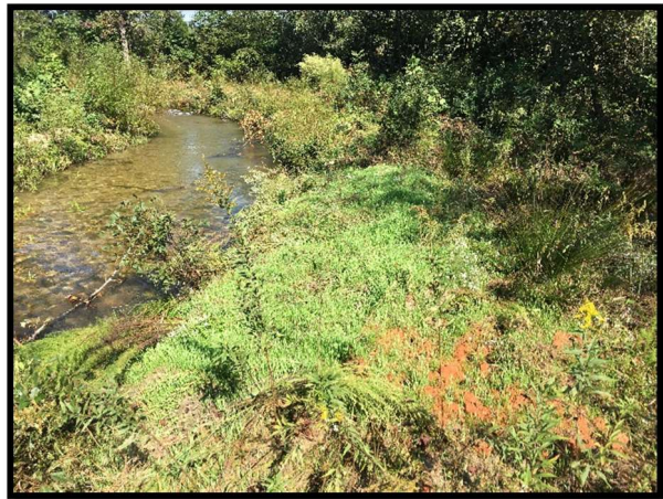
3.21 Repair at station 12+69-12+91
