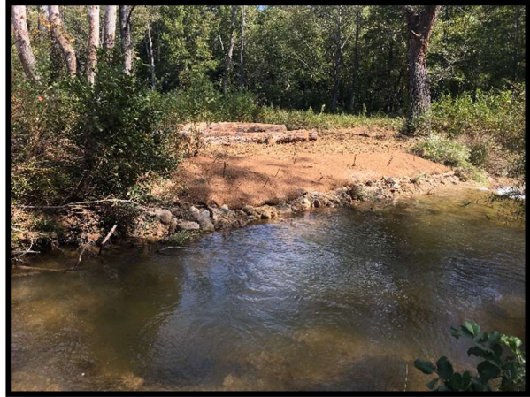
3.25 Repair of erosion at station 37+10-37+30 and relocation of rock step
