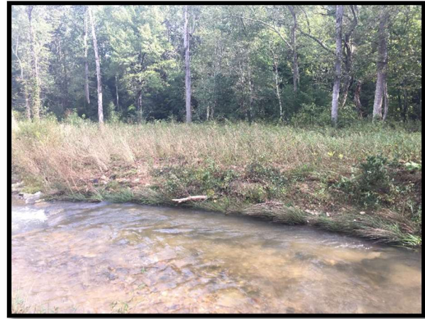
3.27 Repair at station 39+26-39+44
