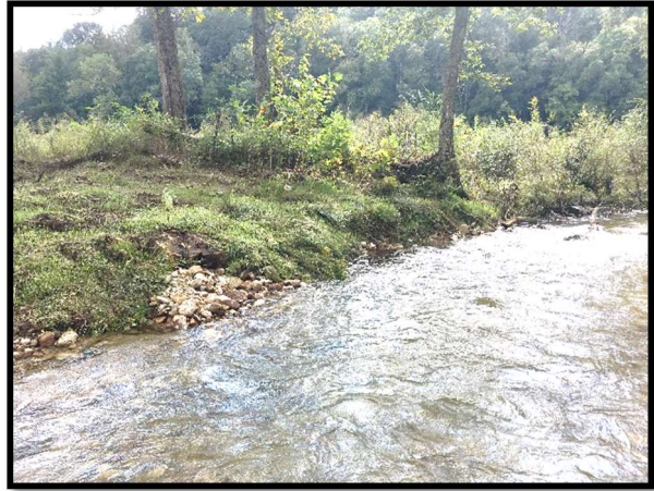
3.19 Repair at station 10+91-11+25
