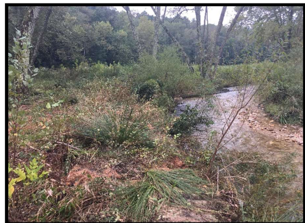
3.23 Repair at station 35+90-36+18
