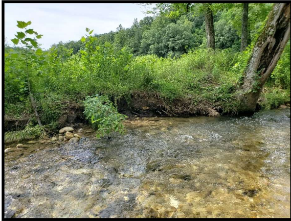
3.18 Erosion at station 10+91-11+25
