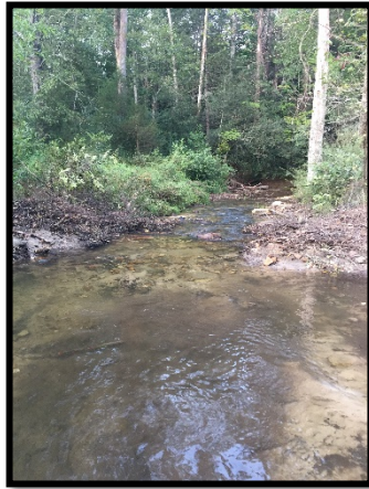
3.5 Beaver dam removal near STA 41+25
