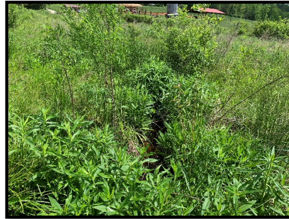
3.6 UT 2 dense bank vegetation STA 10+75
