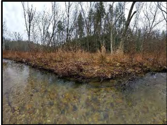
3.25 Minor Erosion at station 40+00.
