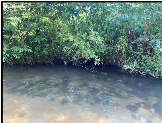
3.21 Moderate toe erosion at station 32+32-32+70. Looking perpendicular.
