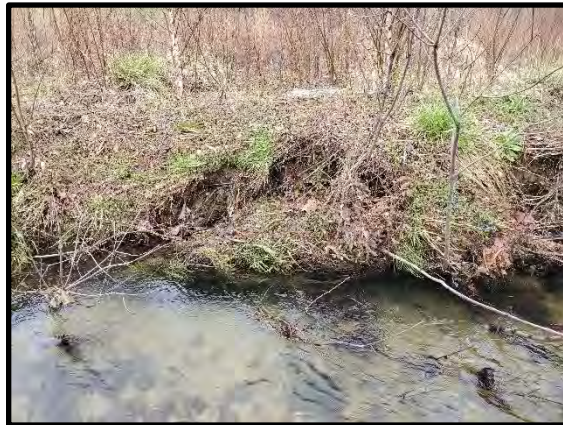
3.20 Mass wasting at station 27+94 – 28+09
