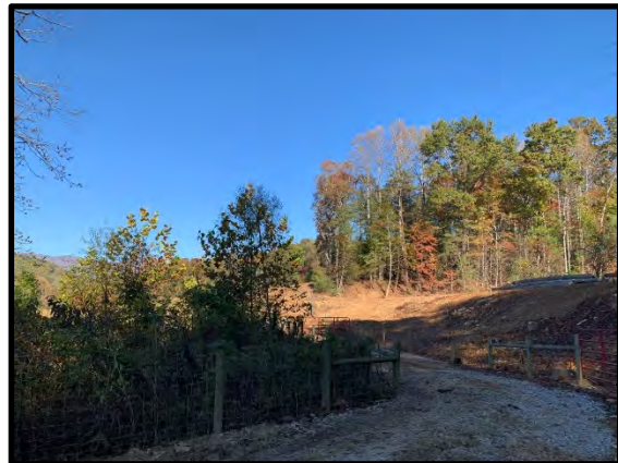
3.28 UT 1 Powerline relocation October 2022
