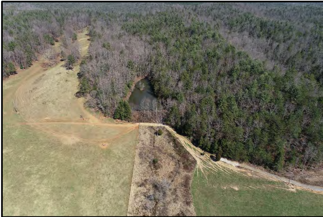
3.31 Pond above UT1 aerial (March 3, 2022)
