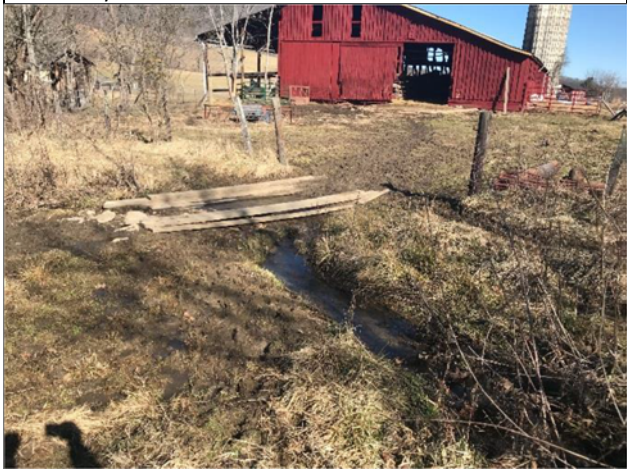
Photo 3: Looking at RHB-1 at an existing crossing near the barn.
