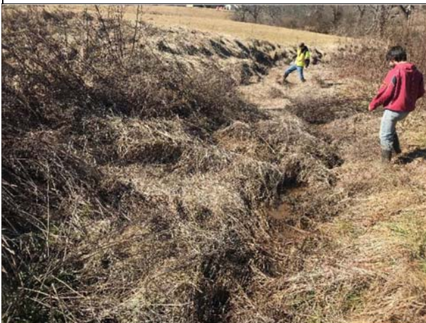
Photo 11: Looking downstream at the start of T2 just south of the Green Valley Road crossing.
