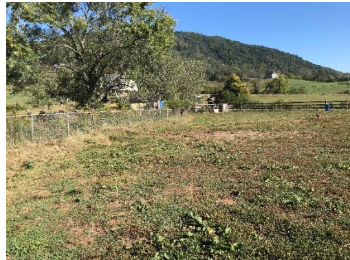
RHB-1 as it nears the confluence with T1; straightened stream is to left of fence and spoil is blocking overland flow on right of fence.
