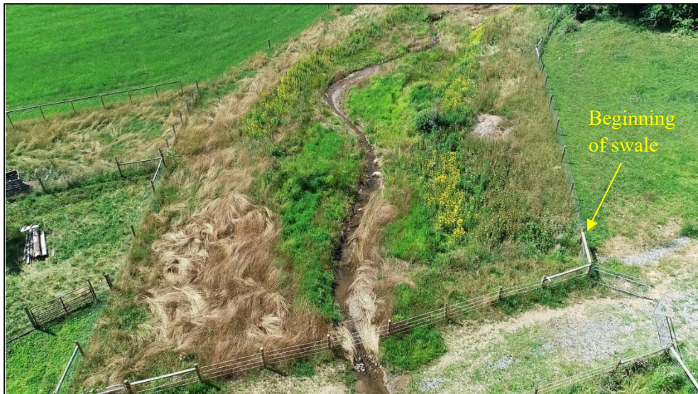
Diversion swale on RHB – MY-01 – 10/10/22
