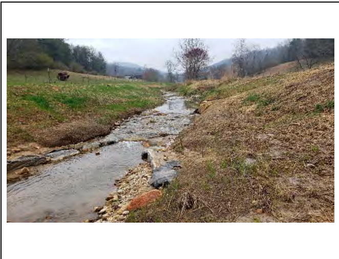
PP-75: Reach 4, view upstream at Station 23+20
