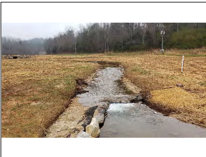
PP-17: Reach 1, view upstream at Station 24+20
