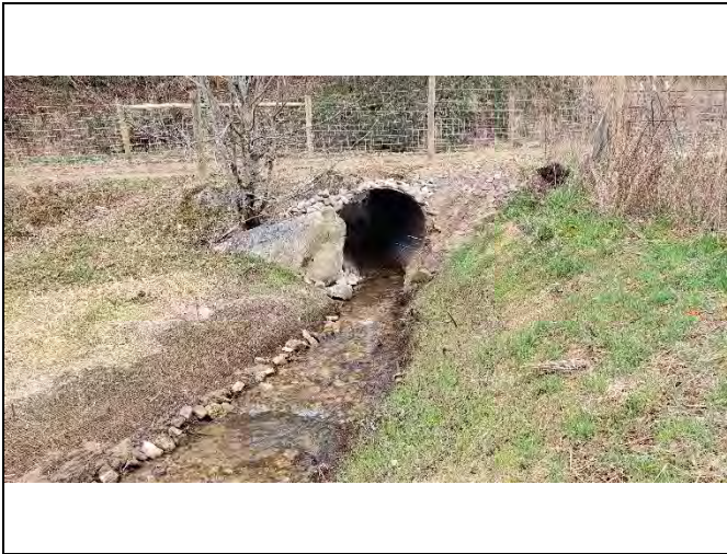
PP-57: Reach 7B, view downstream at Station 33+00
