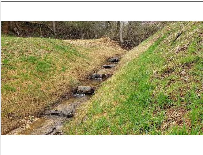
PP-69: Reach 27, view upstream at Station 11+60
