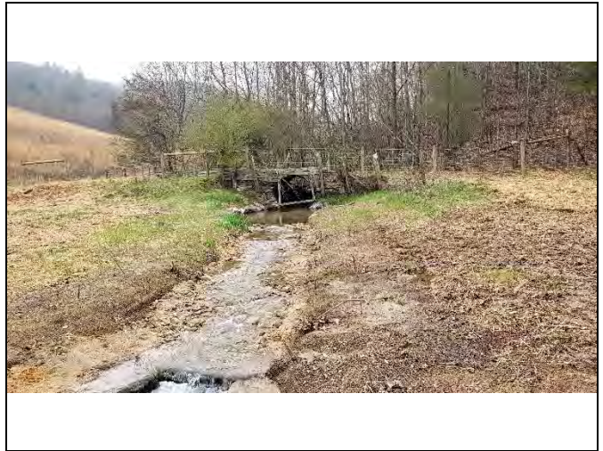
PP-62: Reach 9, view upstream at Station 39+20
