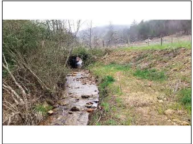
PP-50: Reach 7B, view upstream at Station 25+25
