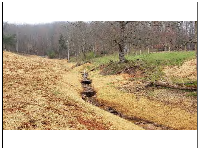
PP-24: Reach 11, view upstream at Station 14+50
