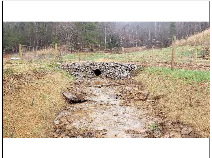
PP-46: Reach 19, view upstream at Station 13+20
