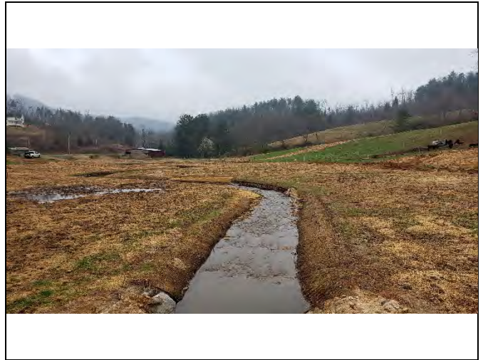
PP-14: Reach 1, view downstream at Station 20+75
