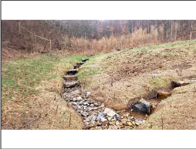
PP-43: Reach 19, view upstream at Station 10+15
