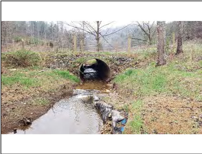
PP-39: Reach 7B, view upstream at Station 22+25
