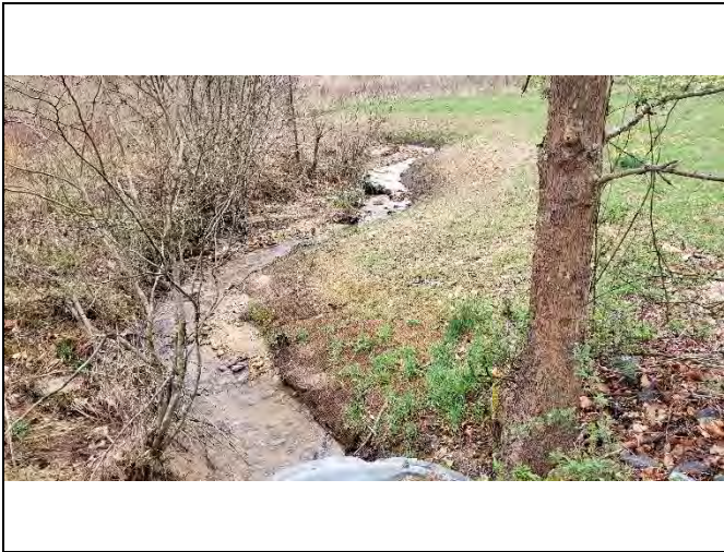
PP-37: Reach 7B, view upstream at Station 21+75
