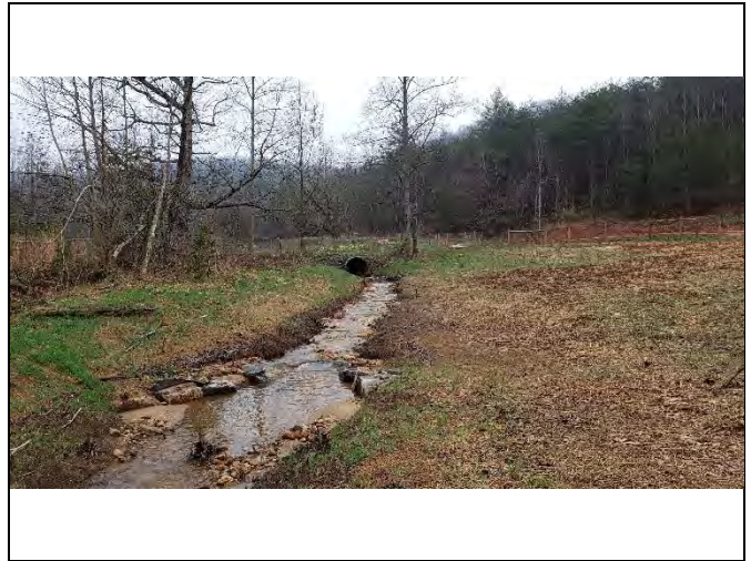
PP-40: Reach 7B, view upstream at Station 23+50
