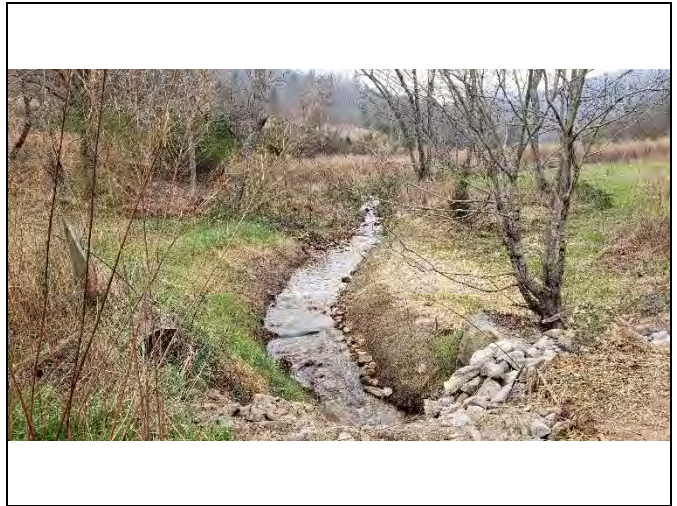
PP-58: Reach 7B, view upstream at Station 33+20
