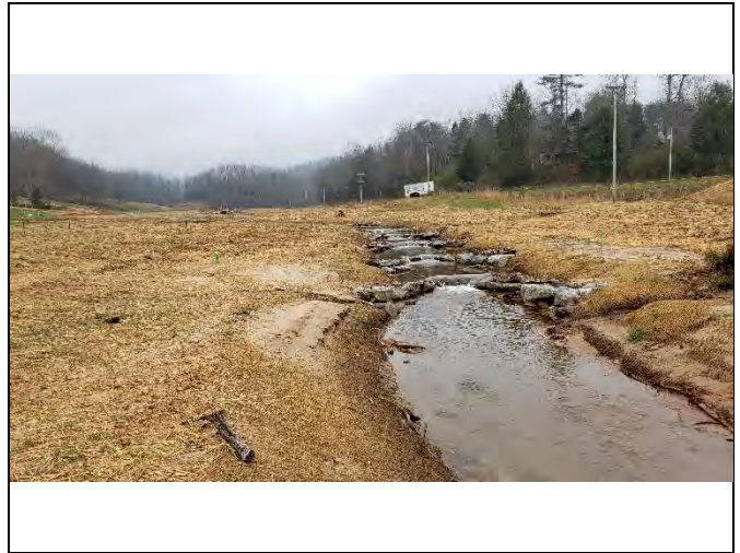
PP-20: Reach 1, view upstream at Station 29+20
