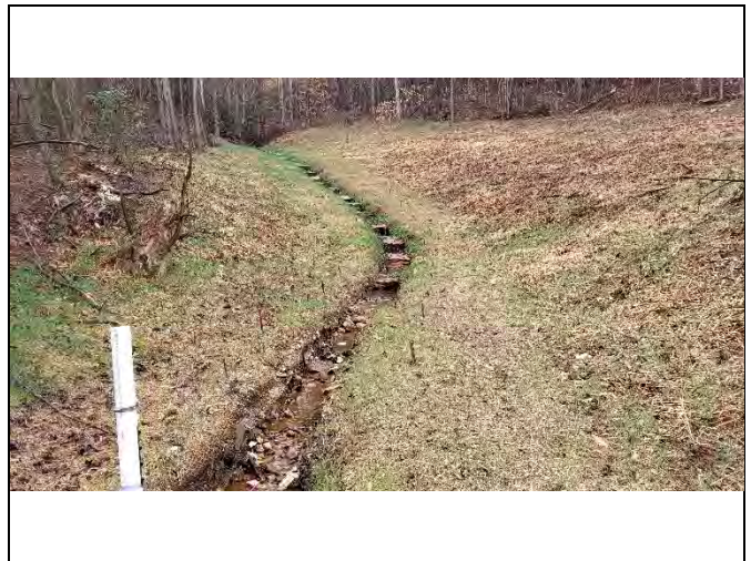
PP-42: Reach 20, view upstream at Station 11+50
