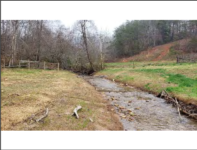
PP-7: Reach 1, view upstream, at Station 10+20
