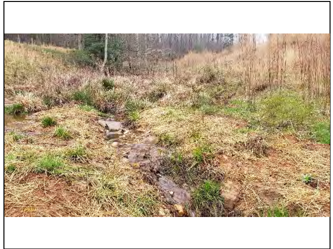
PP-26: Reach 10A, view upstream at Station 12+50
