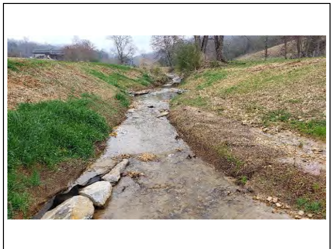
PP-78: Reach 4, view downstream at Station 28+00
