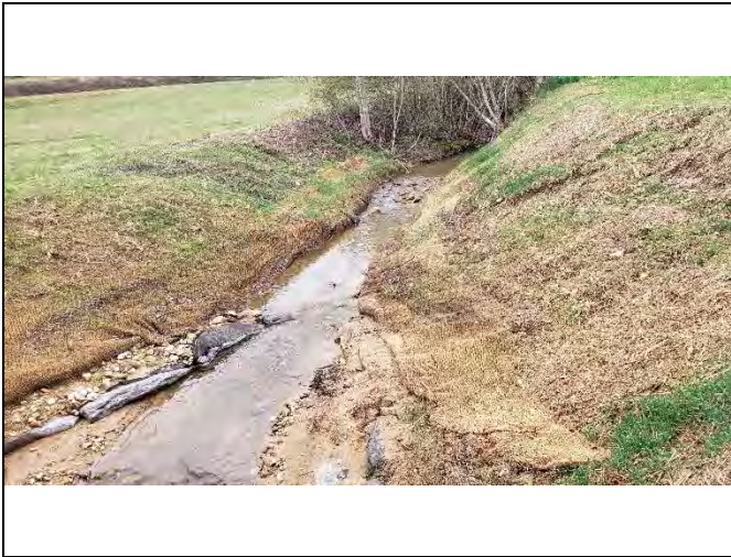
PP-67: Reach 4, view upstream at Station 11+10
