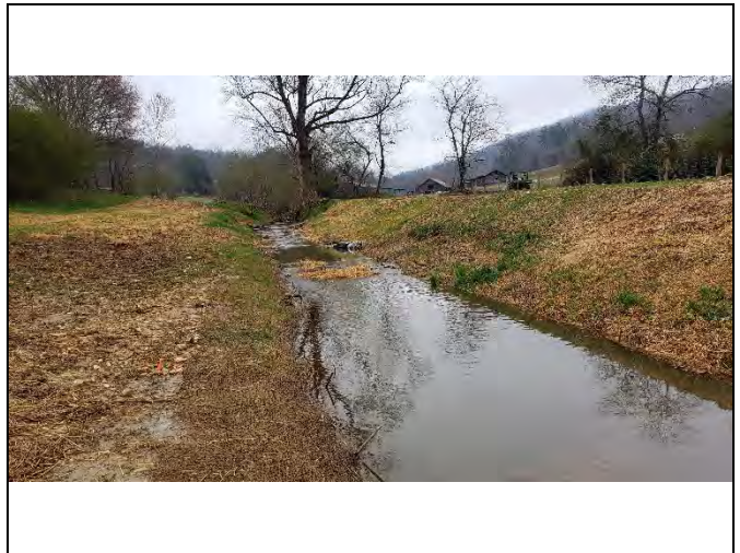
PP-70: Reach 4, view upstream at Station 15+00
