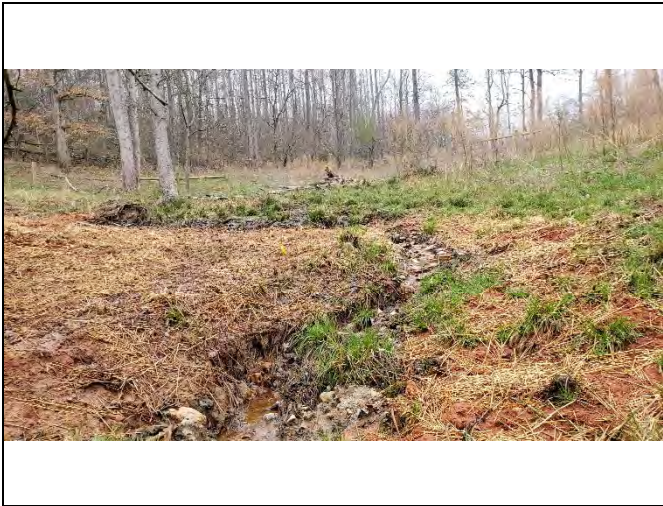
PP-25: Reach 10A, view upstream at Station 10+50
