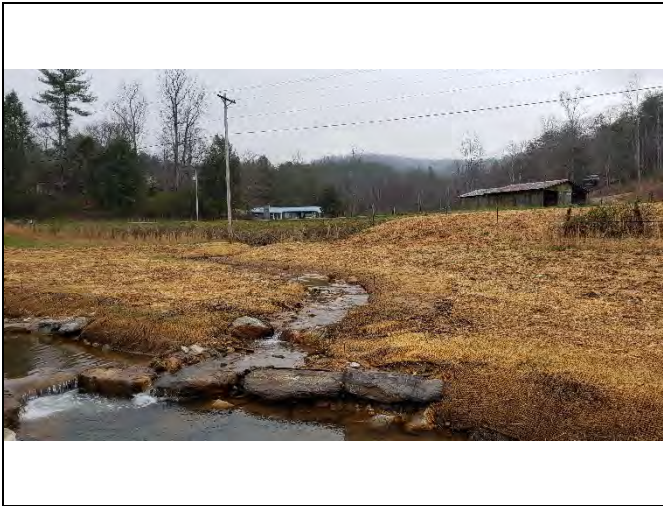
PP-19: Reach 1, view upstream Reach 12 at Station 29+10
