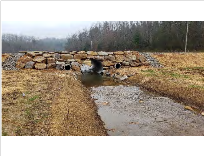
PP-15: Reach 1, view upstream at Station 21+50
