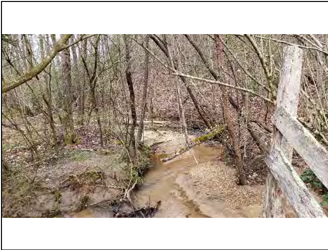
PP-61: Reach 8, view upstream at Station 38+00
