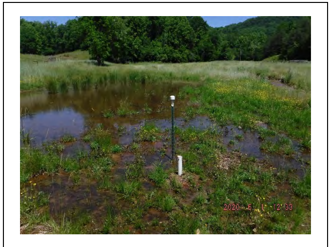
Groundwater Well #3, Reach 1, Station 15+50
