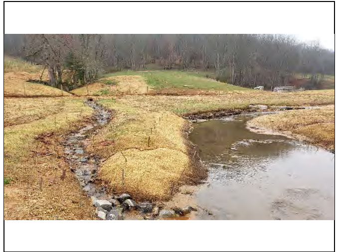
PP-16: Reach 1, confluence of Reach 1 and Reach 11 at Station 22+75
