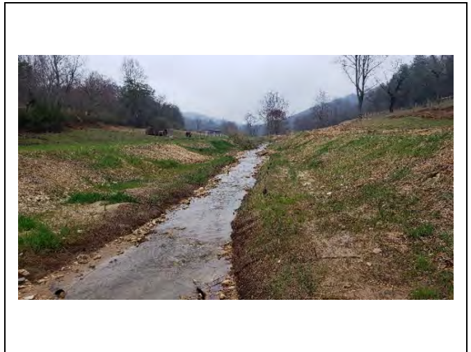
PP-76: Reach 4, view upstream at Station 25+00
