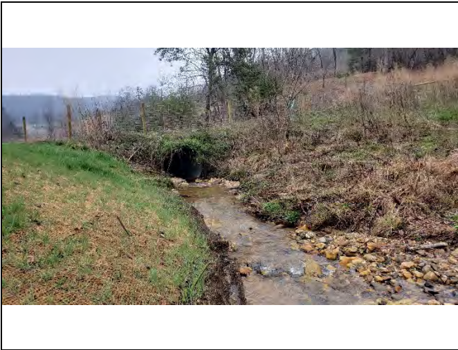
PP-49: Reach 7B, view downstream at Station 24+60
