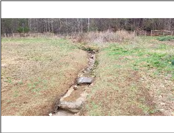
PP-31: Reach 17, view upstream at Station 11+00
