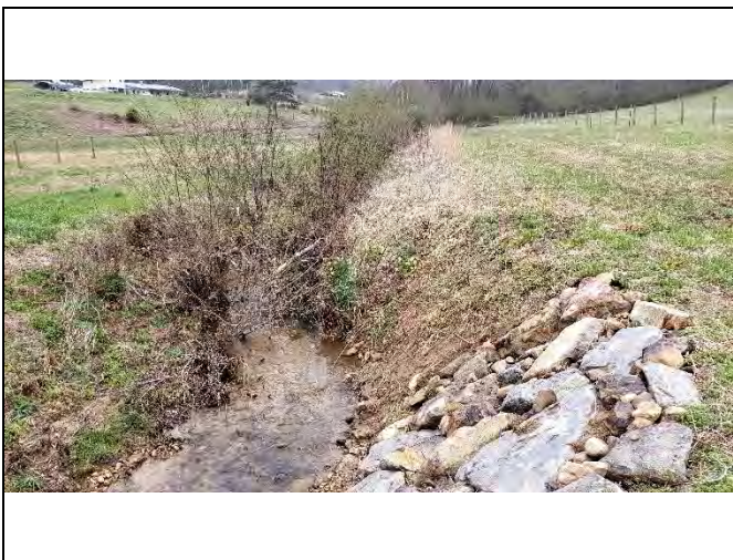
PP-65: Reach 4A, view upstream at Station 13+00
