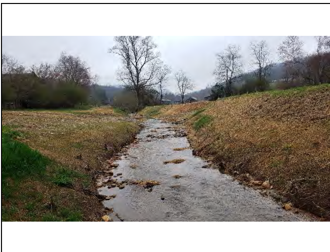
PP-71: Reach 4, view upstream at Station 16+10
