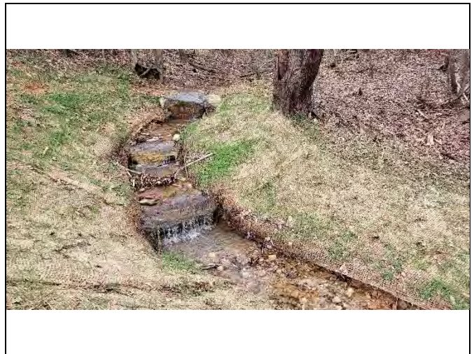
PP-54: Reach 25, view upstream at Station 10+10
