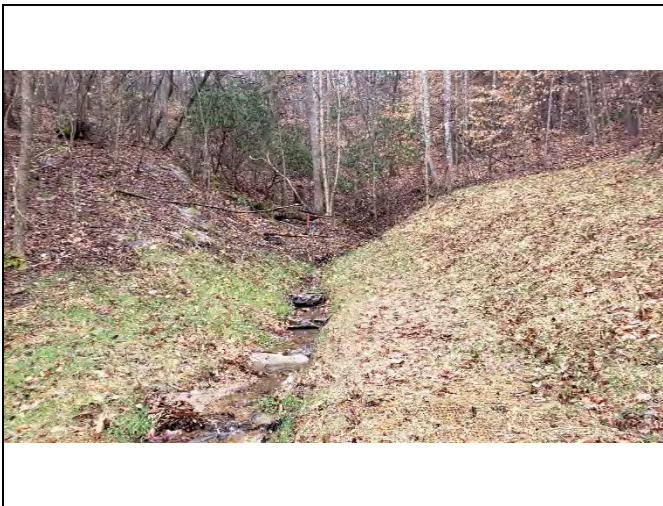
PP-41: Reach 20, view upstream at Station 10+80
