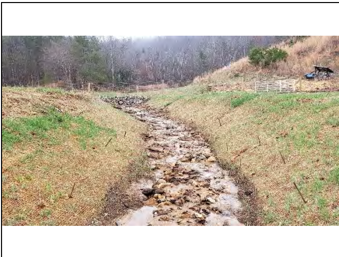
PP-47: Reach 19, view upstream at Station 013+80
