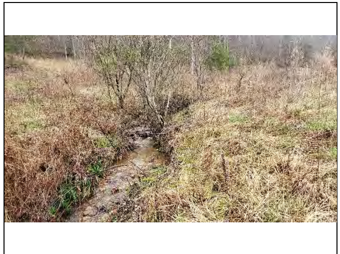
PP-36: Reach 7A, view upstream at Station 20+00
