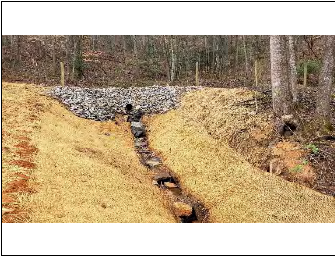
PP-21: Reach 11, view upstream at Station 10+20
