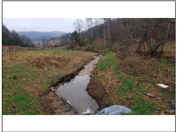
PP-38: Reach 7B, view downstream at Station 22+00
