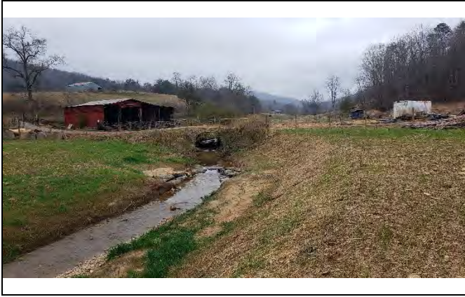
PP-79: Reach 4, view upstream at Station 32+00
