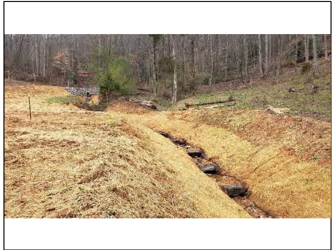
PP-22: Reach 11, view upstream at Station 11+50
