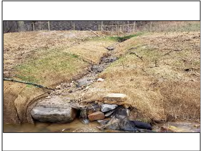
PP-74: Reach 15, view upstream at Station 13+00
