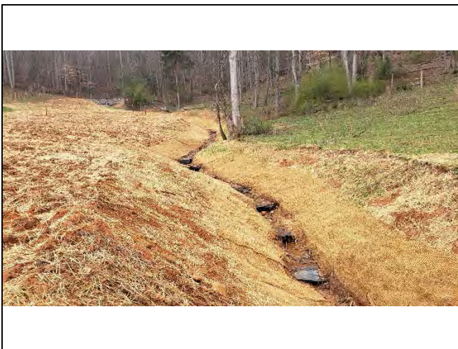
PP-23: Reach 11, view upstream at Station 12+75
