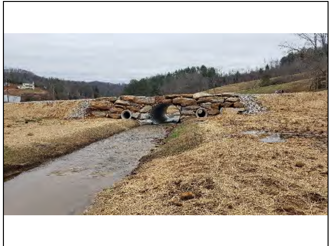
PP-12: Reach 1, view downstream at Station 20+00
