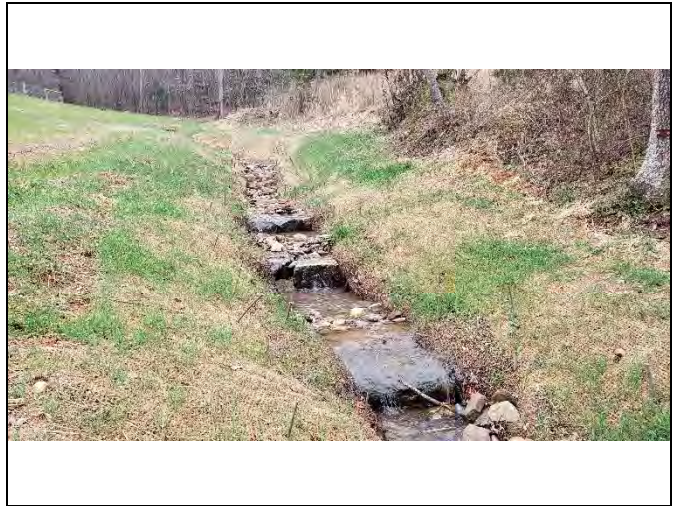
PP-56: Reach 25, view upstream at Station 13+40
