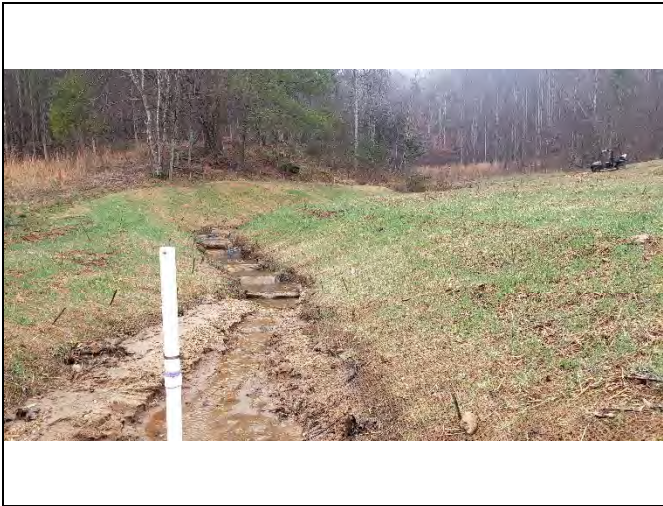
PP-45: Reach 19, view upstream at Station 12+80
