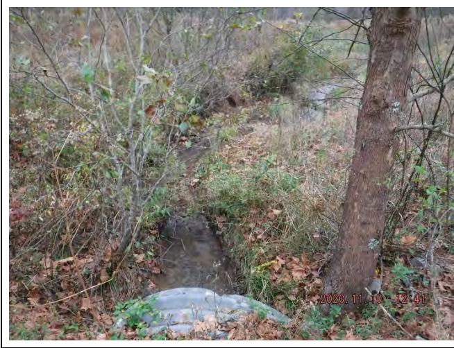
PP-37: Reach 7B, view upstream at Station 21+75. (November 10, 2020)
