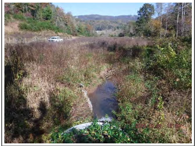
PP-38: Reach7B, view downstream at Station 22+00. (October 21, 2020)
