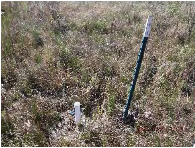
Monitoring Well 7. (November 5, 2020)
