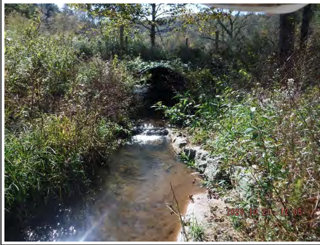
PP-39: Reach 7B, view upstream at Station 22+25. (October 21, 2020)
