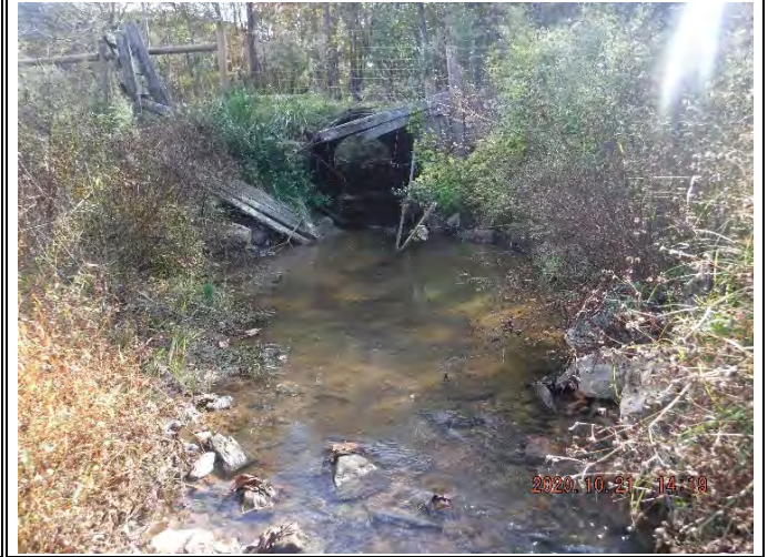
PP-62: Reach 9, view upstream at Station 39+20. (October 21, 2020)
