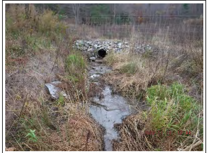
PP-46: Reach 19, view upstream at Station 13+20. (November 10, 2020)
