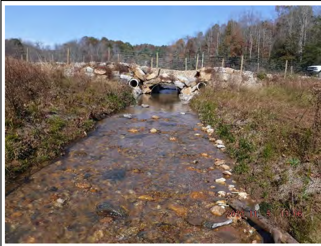
PP-15: Reach 1, view upstream at Station 21+50. (November 5, 2020)
