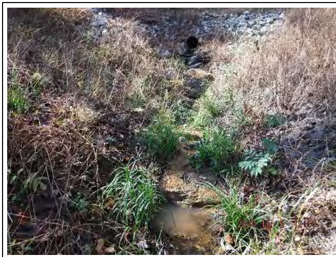
PP-21: Reach 11, view upstream at Station 10+20. (November 5, 2020)
