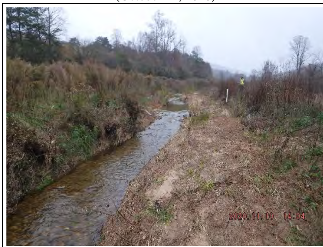
PP-78: Reach 4, view upstream at Station 28+00. (November 10, 2020)
