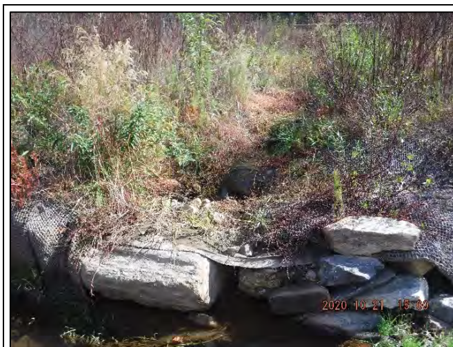
PP-74: Reach 15, view upstream at Station 13+00. (October 21, 2020)
