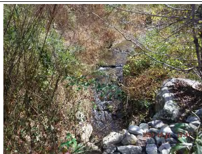
PP-58: Reach 7B, view upstream at Station 33+20. (October 21, 2020)
