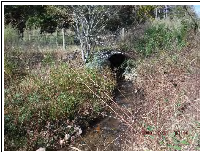
PP-57: Reach 7B, view downstream at Station 33+00. (October 21, 2020)
