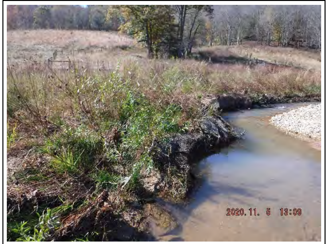
PP-16: Reach 1, confluence of Reach 1 and Reach 11 at Station 22+75. (November 5, 2020)
