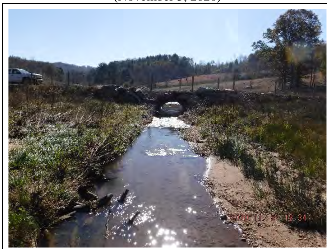
PP-12: Reach 1, view downstream at Station 20+00. (November 5, 2020)
