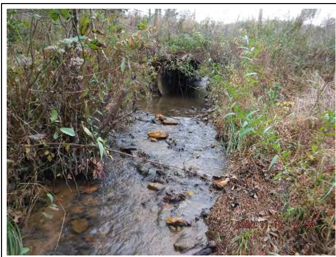
PP-50: Reach 7B, view upstream at Station 25+25. (November 10, 2020)
