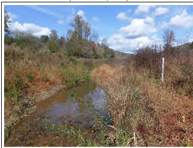
PP-77: Reach 4, view upstream at Station 28+30. (October 21, 2020)
