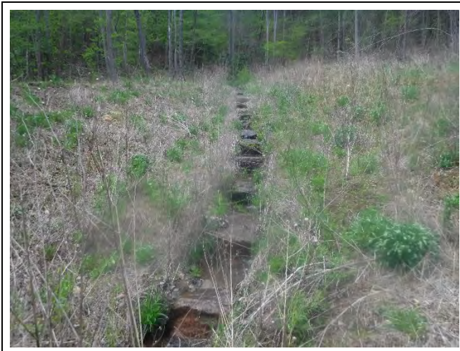
PP-41: Reach 20, view upstream at Station 10+80. (April 15, 2021)
