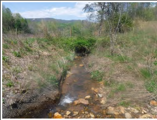
PP-49: Reach 7B, view downstream at Station 24+60. (April 15, 2021)
