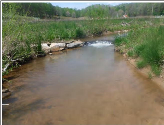
PP-17: Reach 1, view upstream at Station 24+20. (April 15, 2021)
