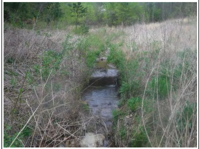
PP-44: Reach 19, view upstream at Station 11+85. (April 15, 2021)
