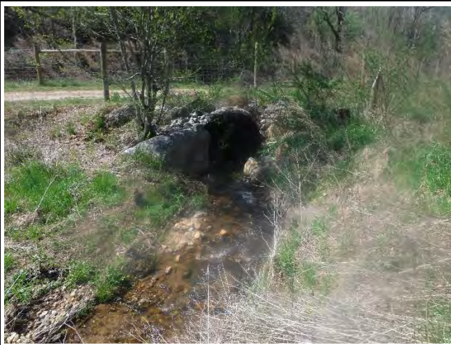
PP-57: Reach 7B, view downstream at Station 33+00. (April 15, 2021)
