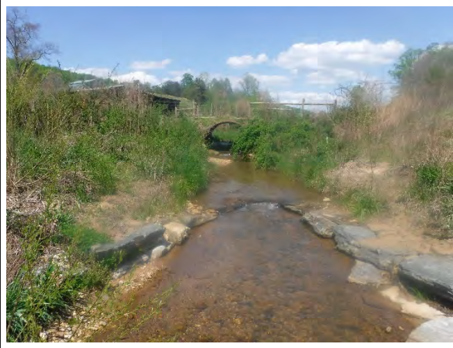
PP-79: Reach 4, view upstream at Station 32+00. (April 15, 2021)
