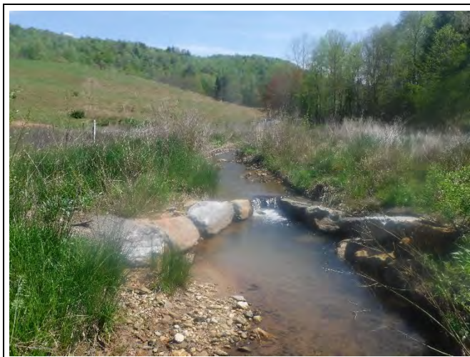
PP-63: Reach 9, view upstream at Station 41+00. (April 15, 2021)
