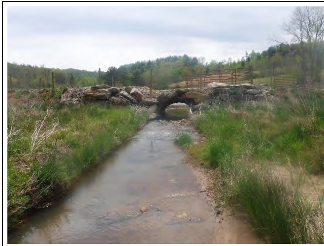
PP-12: Reach 1, view downstream at Station 20+00. (April 15, 2021)
