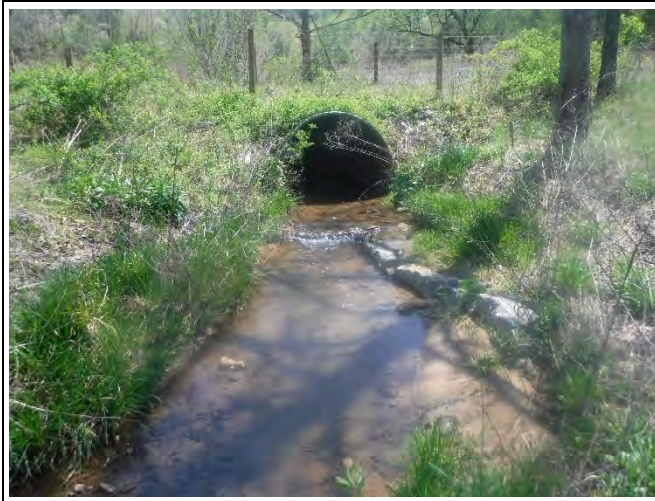
PP-39: Reach 7B, view upstream at Station 22+25. (April 15, 2021)
