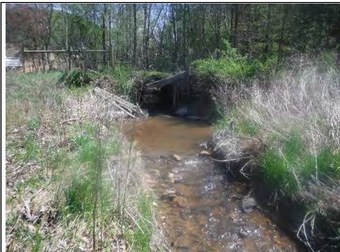
PP-62: Reach 9, view upstream at Station 39+20. (April 15, 2021)
