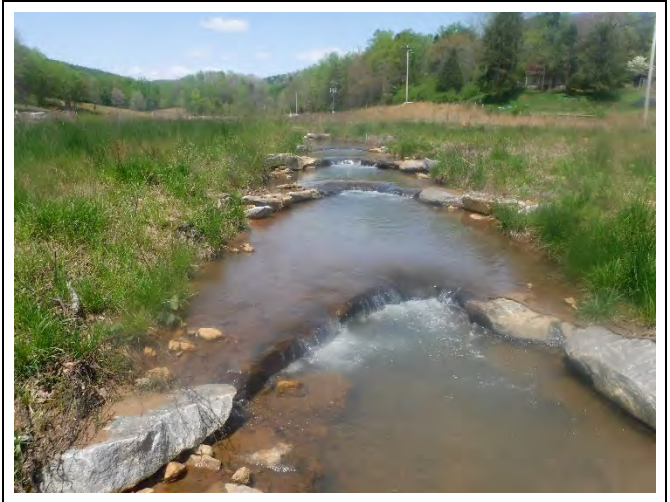
PP-20: Reach 1, view upstream at Station 29+20. (April 15, 2021)
