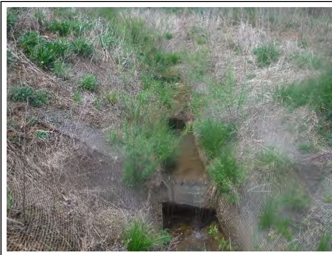
PP-23: Reach 11, view upstream at Station 12+75. (April 15, 2021)
