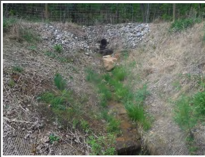
PP-21: Reach 11, view upstream at Station 10+20. (April 15, 2021)
