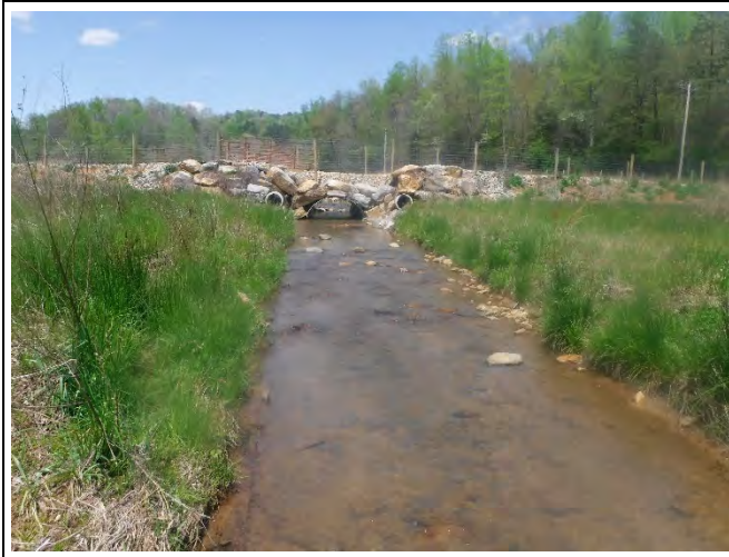
PP-15: Reach 1, view upstream at Station 21+50. (April 15, 2021)
