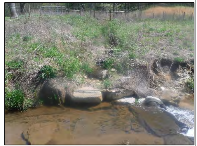
PP-74: Reach 15, view upstream at Station 13+00. (April 15, 2021)
