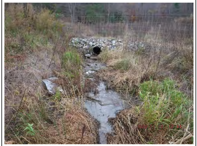
PP-46: Reach 19, view upstream at Station 13+20. (April 15, 2021)
