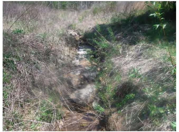
PP-56: Reach 25, view upstream at Station 13+40. (April 15, 2021)
