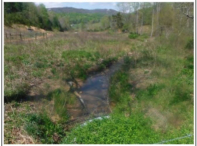
PP-38: Reach 7B, view downstream at Station 22+00. (April 15, 2021)
