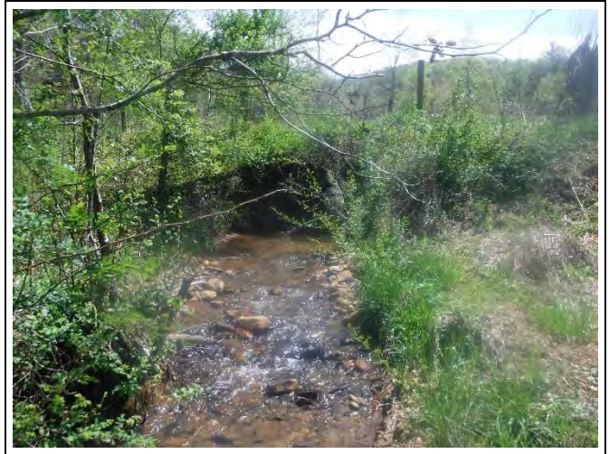
PP-50: Reach 7B, view upstream at Station 25+25. (April 15, 2021)
