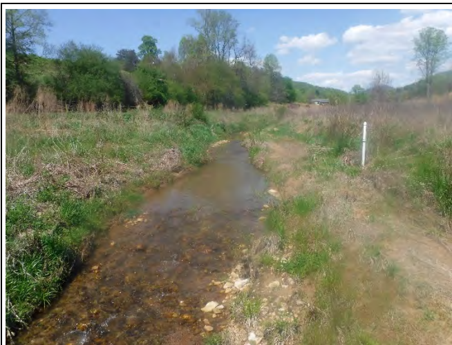
PP-77: Reach 4, view upstream at Station 28+30. (April 15, 2021)
