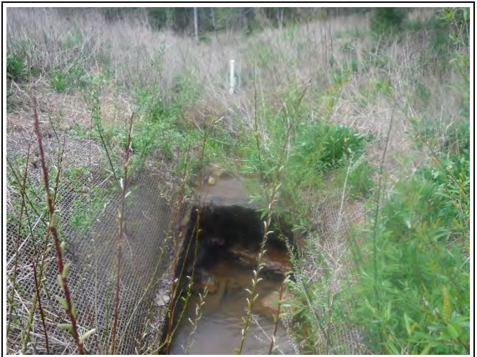
PP-24: Reach 11, view upstream at Station 14+50. (April 15, 2021)
