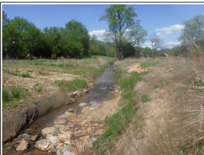
PP-71: Reach 4, view upstream at Station 16+10. (April 15, 2021)
