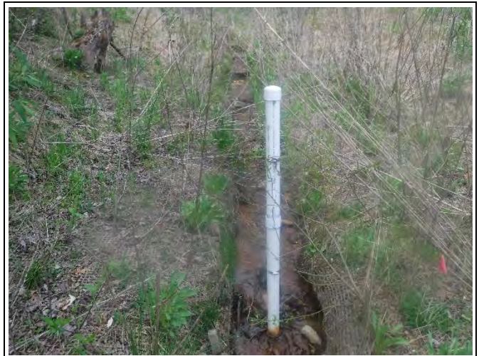
PP-42: Reach 20, view upstream at Station 11+50. (April 15, 2021)
