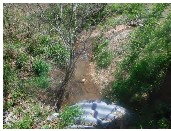
PP-37: Reach 7B, view upstream at Station 21+75. (April 15, 2021)
