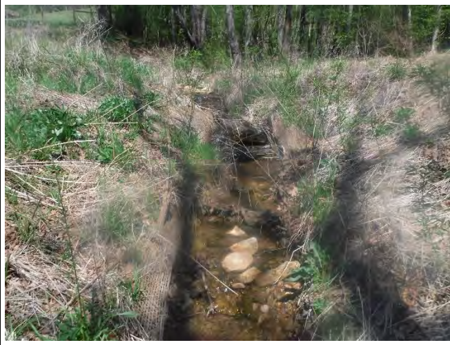
PP-55: Reach 25, view upstream at Station 11+20. (April 15, 2021)
