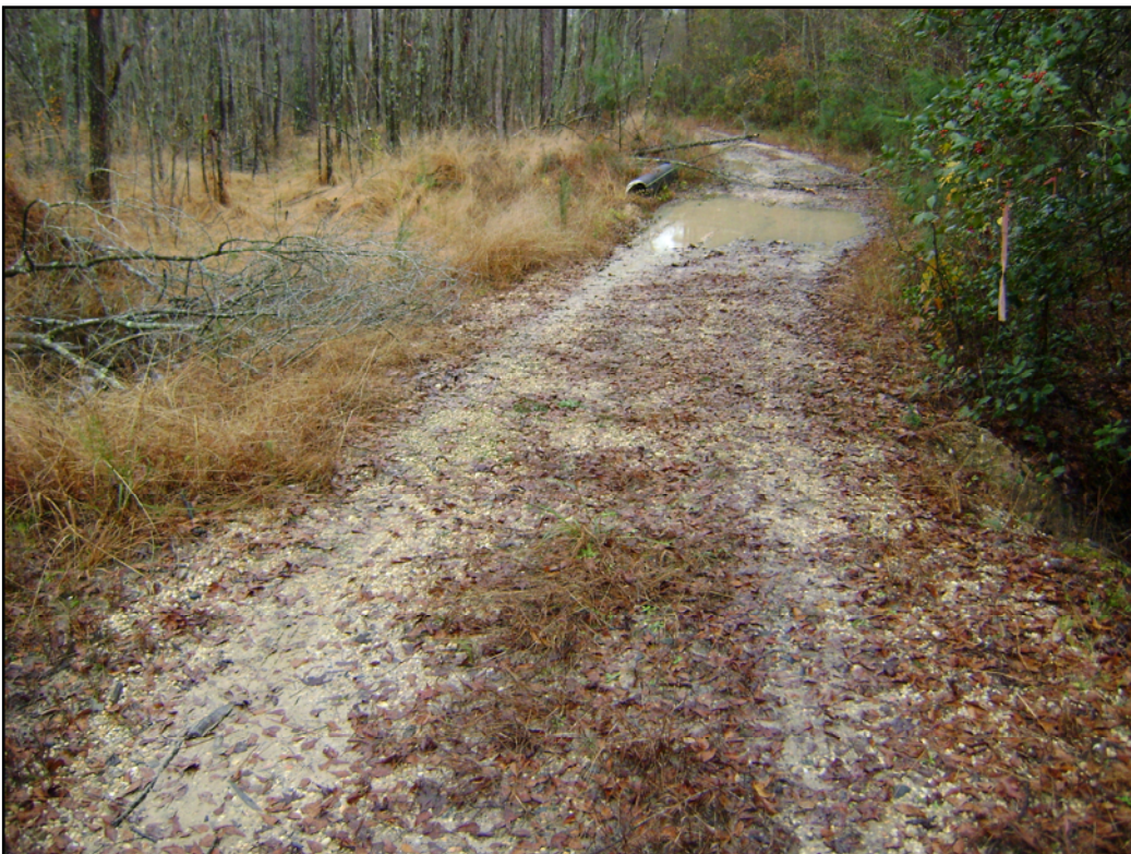
Road with culverts installed - November 23, 2009.
