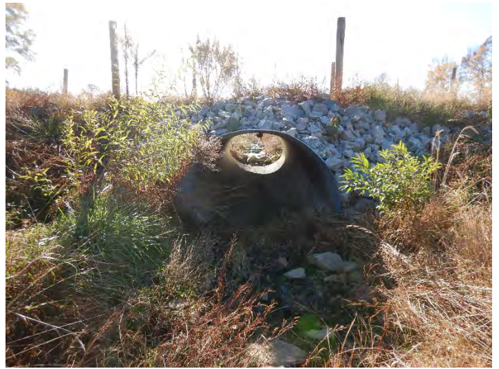
CULVERT CROSSING Sandy Branch R1 – downstream (11/19/2021)
