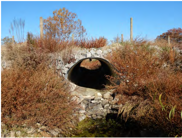
CULVERT CROSSING Sandy Branch R1 – upstream (11/19/2021)
