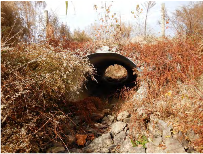
Sandy Branch R1 – Looking Upstream (11/20/2023)
