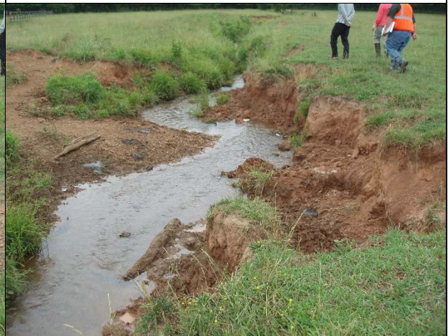
View looking south and downstream at T1. Significant bank erosion has been caused by cattle access to the stream. 6/4/15
