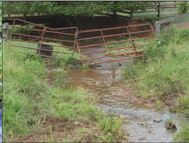
View looking north and upstream at the eroded stream entering Tributary 1 (T1) after flowing under a bridge for cattle crossing. 6/4/15
