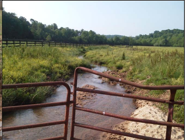
View looking south and downstream at the straightened stream channel at the top of the project reach. 6/4/2015.
