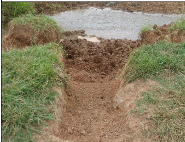
View looking east at erosion from cattle access to T1. 6/4/15
