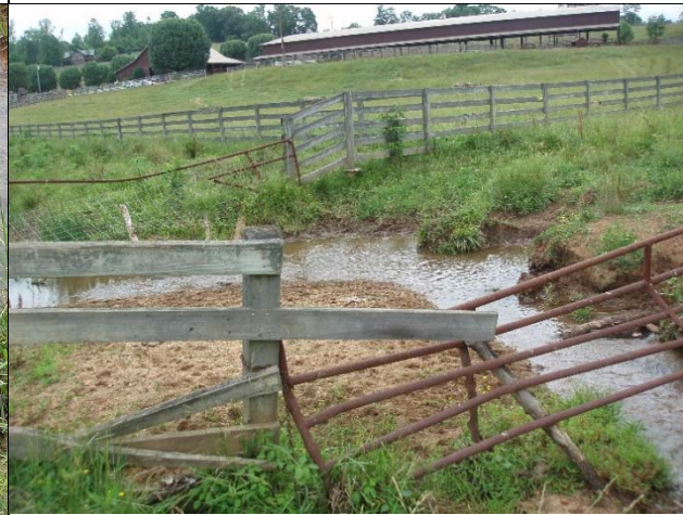
View looking northeast and upstream at the top of T1. 6/4/15
