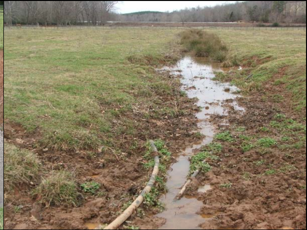
Ditches that drain the site will be filled to increase hydrology and the connection between the stream and wetlands on site. 2/12/2013.
