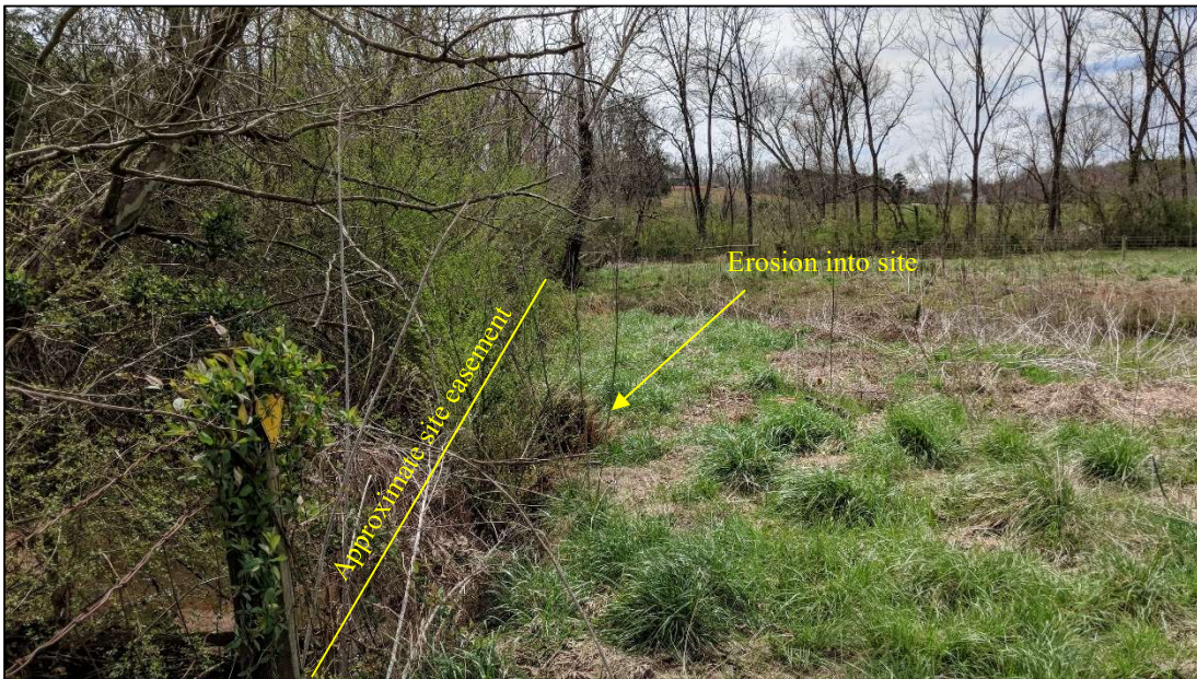
Photo 4. View along easement boundary where stream bank is eroding, 8/29/2018
