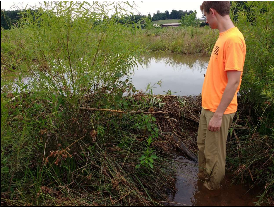
Photo 1. One of the beaver dams onsite (has been removed), 6/28/18
