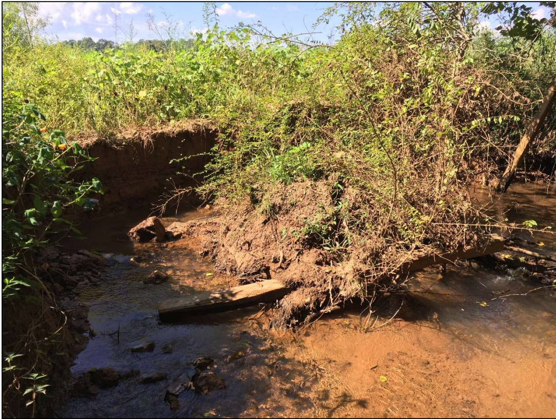
Photo 3. Eroding stream bank that is encroaching into easement, 8/29/2018
