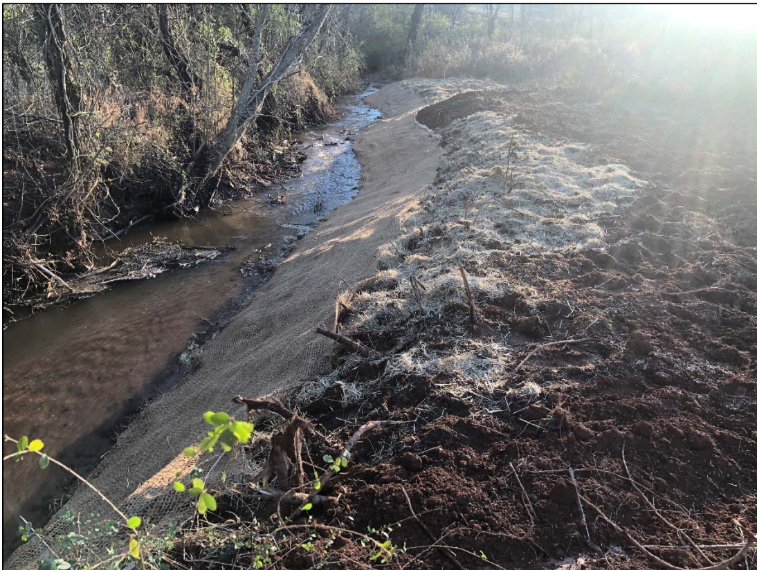
Photo 2. Stream bank after repair, 11/21/2019
