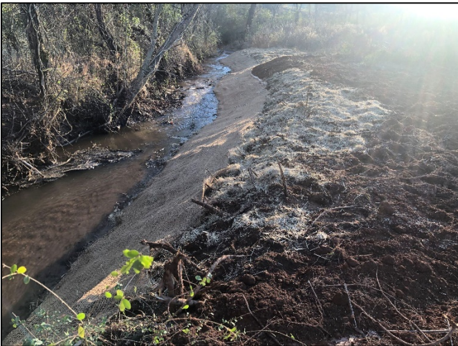
11/21/19 – Immediately after repair
