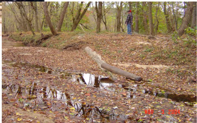
November 3, 2004 Sandy Creek Stream Enhancement Log Vanes
