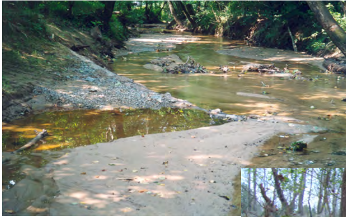
Log Vane #7, Station 15 + 39 July 12, 2003
