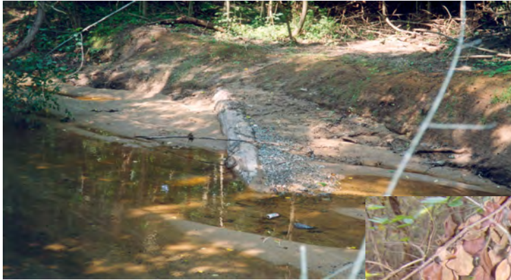
Log Vane # 9, Station 19 +72
