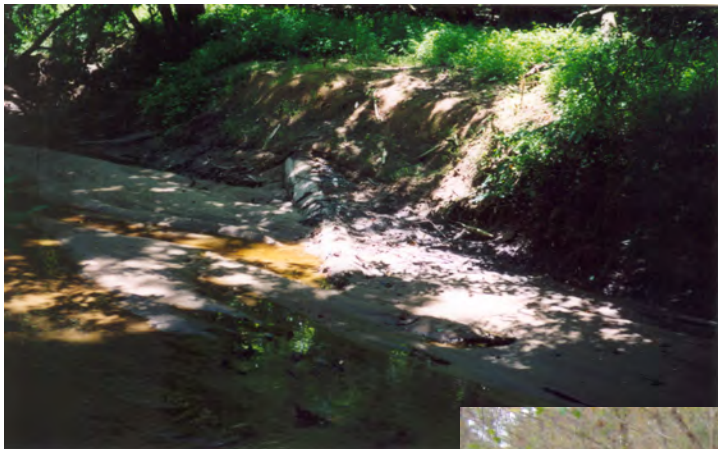
Log Vane #10, Station 20 + 91
