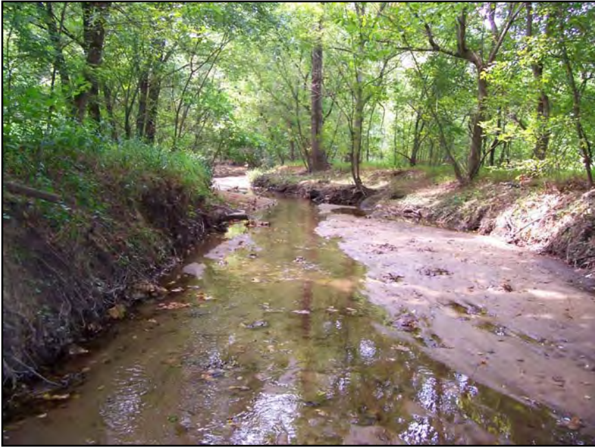
Photo Station 3: Log Vane #3 (Station 6 + 55)
