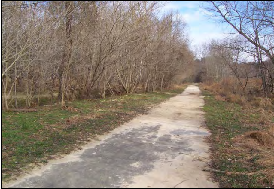
Photo 1. Sediment layer covering adjacent greenway path after a bankfull event
