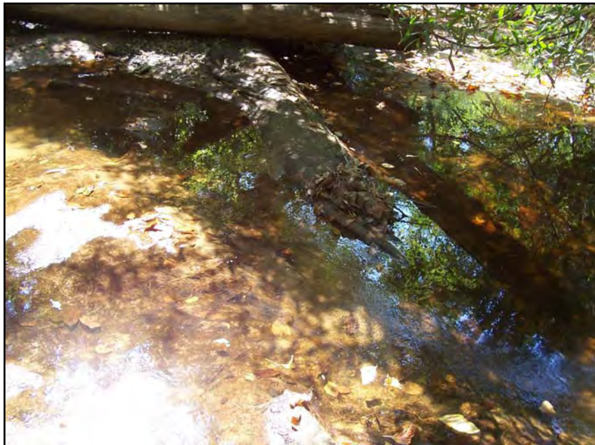
Photo L12: Log Vane 12 at Station 24 + 20 (August 21, 2007)
