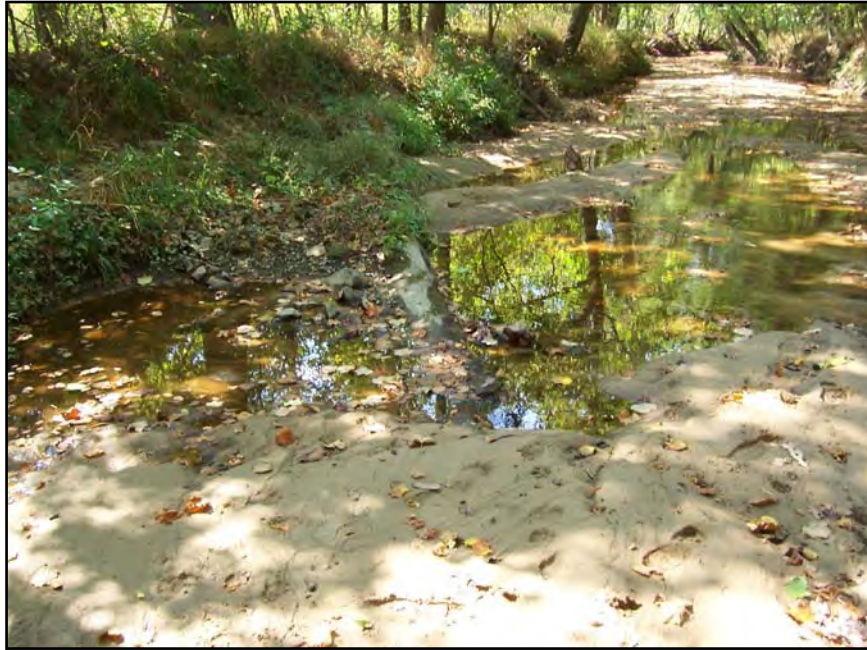
Photo L7: Log Vane 7 at Station 15 + 39 (August 21, 2007)
