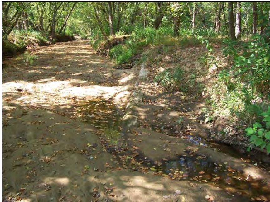
Photo L4: Log Vane 4 at Station 8 + 88 (August 21, 2007)
