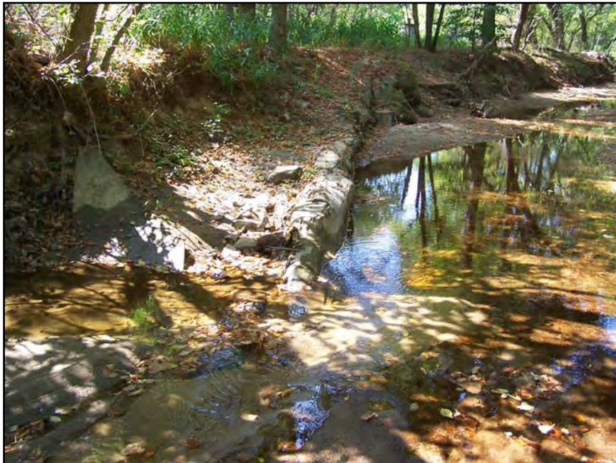
Photo L2: Log Vane 2 at Station 4 + 12 (August 21, 2007)
