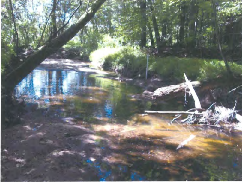
Photo Station 1: Log Vane #1 (Station 2 + 04)
