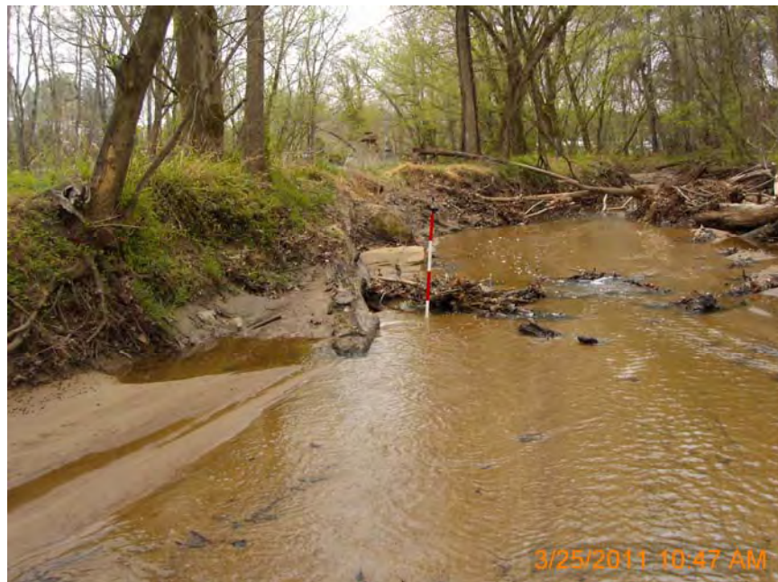
Woody debris obstruction
