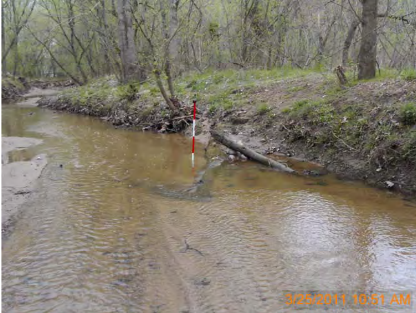
Photo Station 3: Log Vane #3 (Station 6 + 55)
