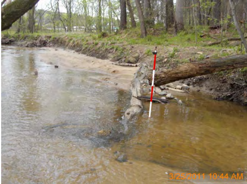
Photo Station 1: Log Vane #1 (Station 2 + 04)
