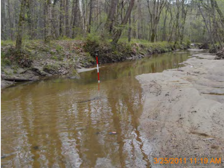
Photo Station 13: Log Vane #13 (Station 26 + 12)
