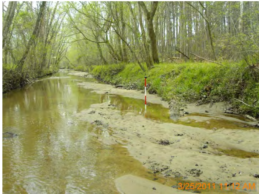
Photo Station 10: Log Vane #10 (Station 20 + 91)
