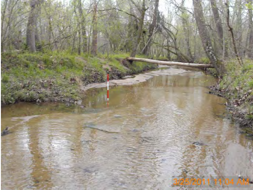
Photo Station 7: Log Vane #7 (Station 15 + 39)
