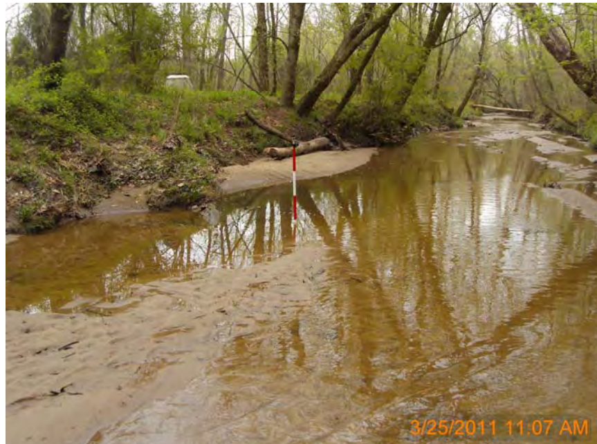
Photo Station 8: Log Vane #8 (Station 17 + 45)
