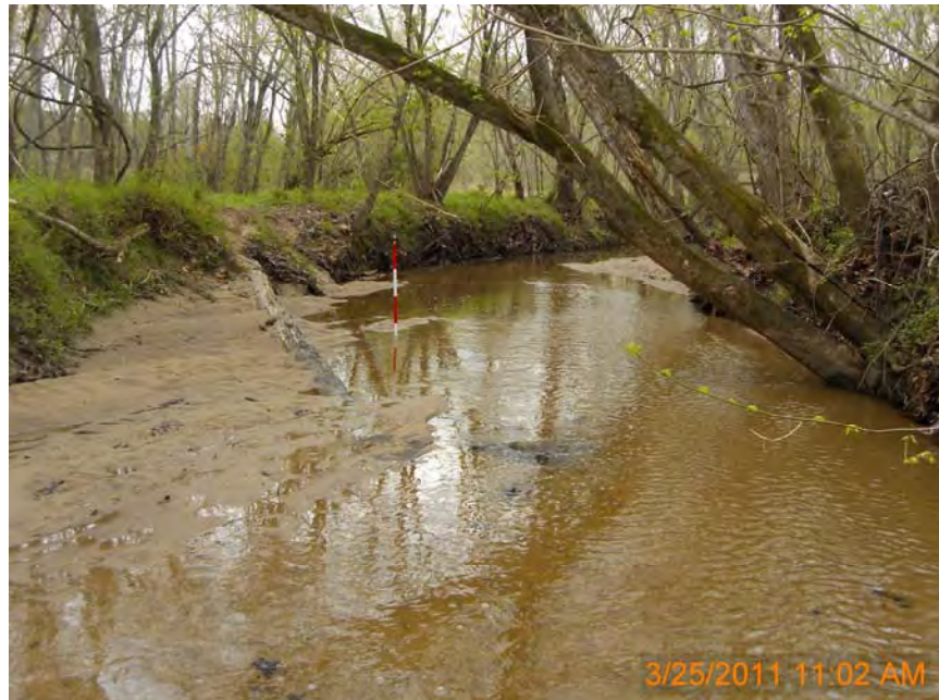
Photo Station 6: Log Vane #6 (Station 13 + 83)
