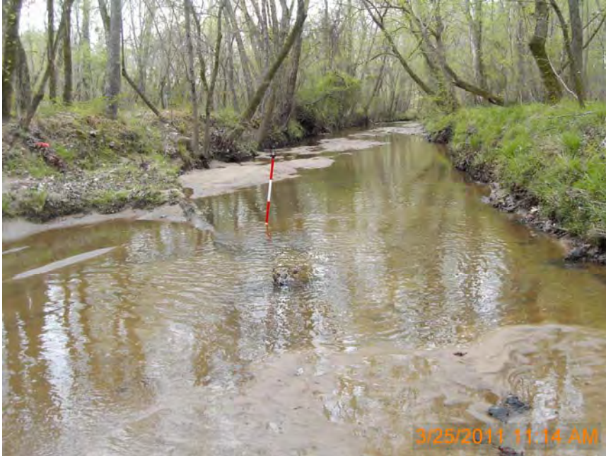
Photo Station 11: Log Vane #11 (Station 22 + 66)
