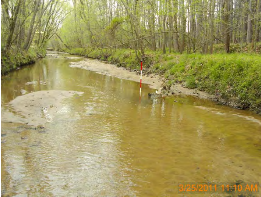
Photo Station 9: Log Vane #9 (Station 19 + 72)
