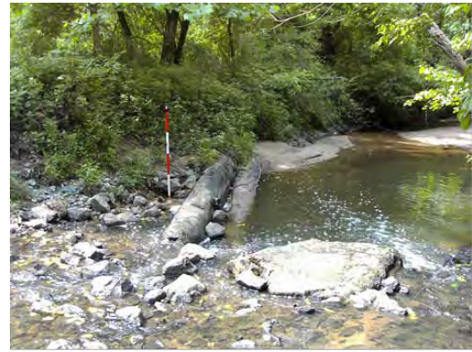
Photo Station 5: Log Vane #5 (Station 10+99)
