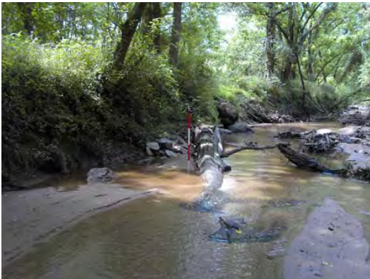
Photo Station 2: Log Vane #2 (Station 4+12)
