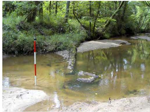
Photo Station 11: Log Vane #11 (Station 22+66)
