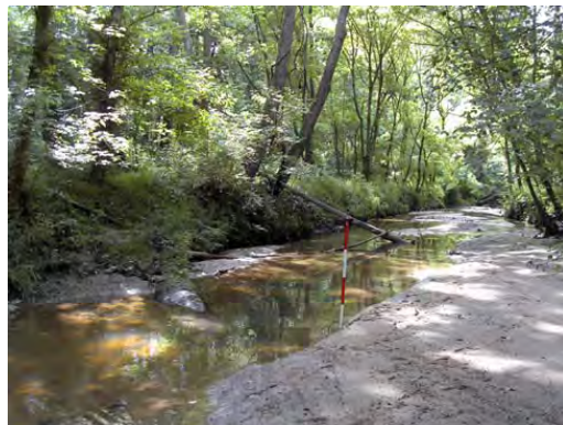
Photo Station 13: Log Vane #13 Station (26 + 12)
