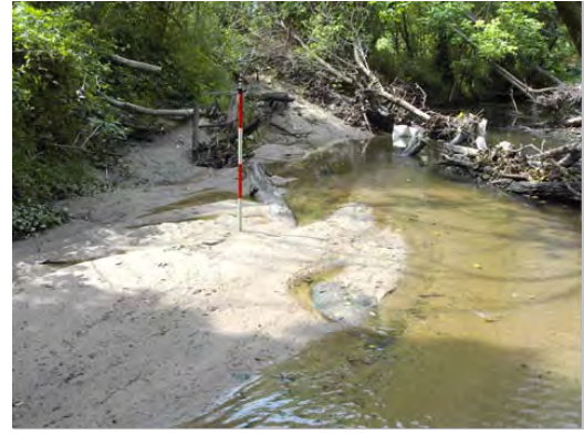
Photo Station 6: Log Vane #6 (Station 13+83)
