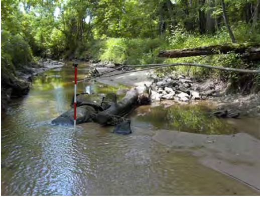
Photo Station 1: Log Vane #1 (Station 2+04)
