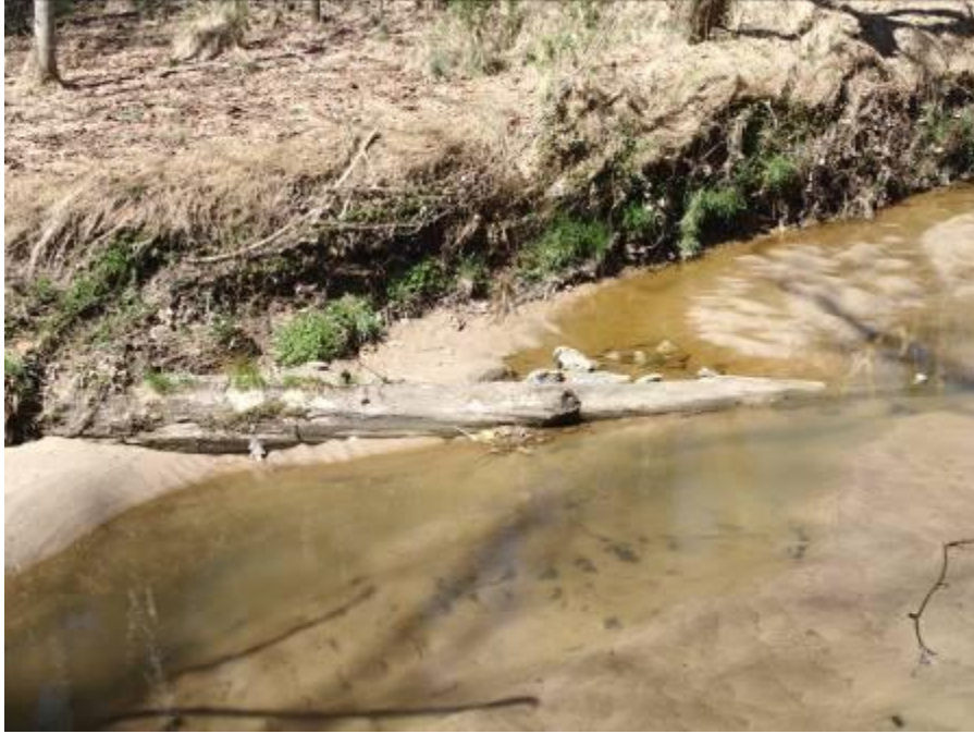
Station 19+72. Upstream facing view of log vane from left descending bank.
