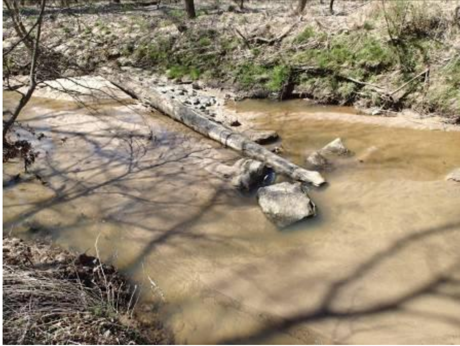
Stion 6+55. Downstream facing view of log vane from descending bank.
