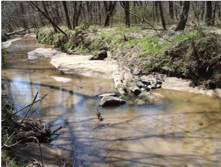
Station 8+88. Downstream facing view of log vane from left descending bank.
