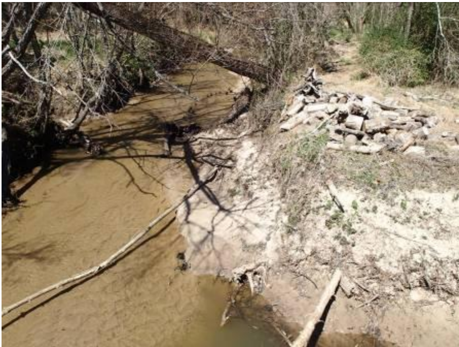
Station 0+00. Upstream facing view from 15-501 culvert.
