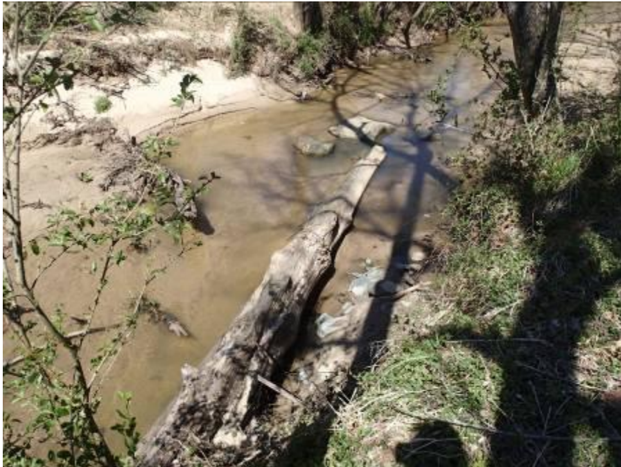
Station 4+12. Upstream facing view of log vane from left descending bank.
