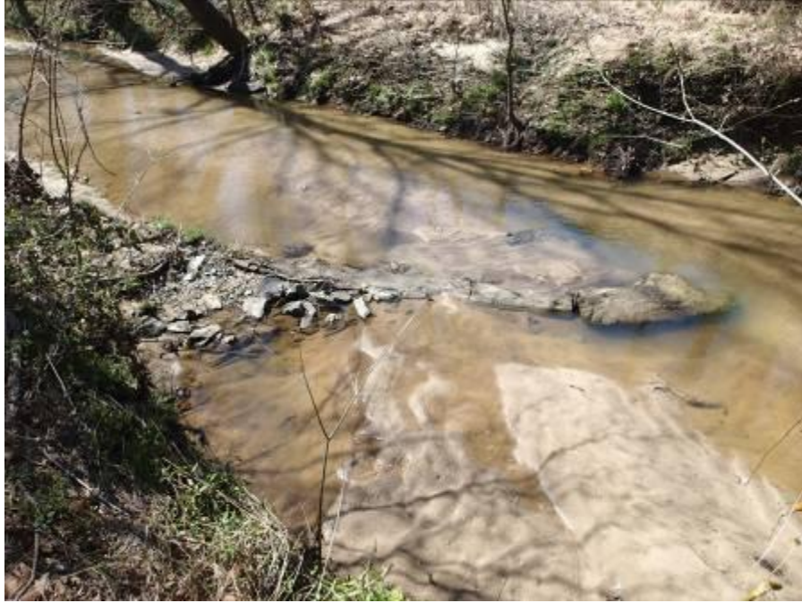
Station 15+39. Downstream facing view of log vane from left descending bank.
