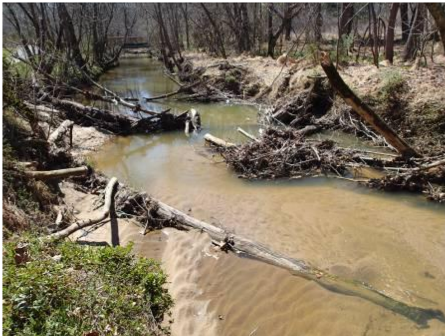
Station 13+83. Downstream facing view of log vane from left descending bank.
