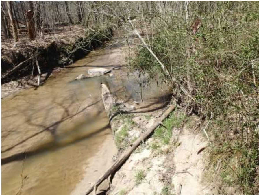
Station 24+20. Upstream facing view of log vane from left descending bank.
