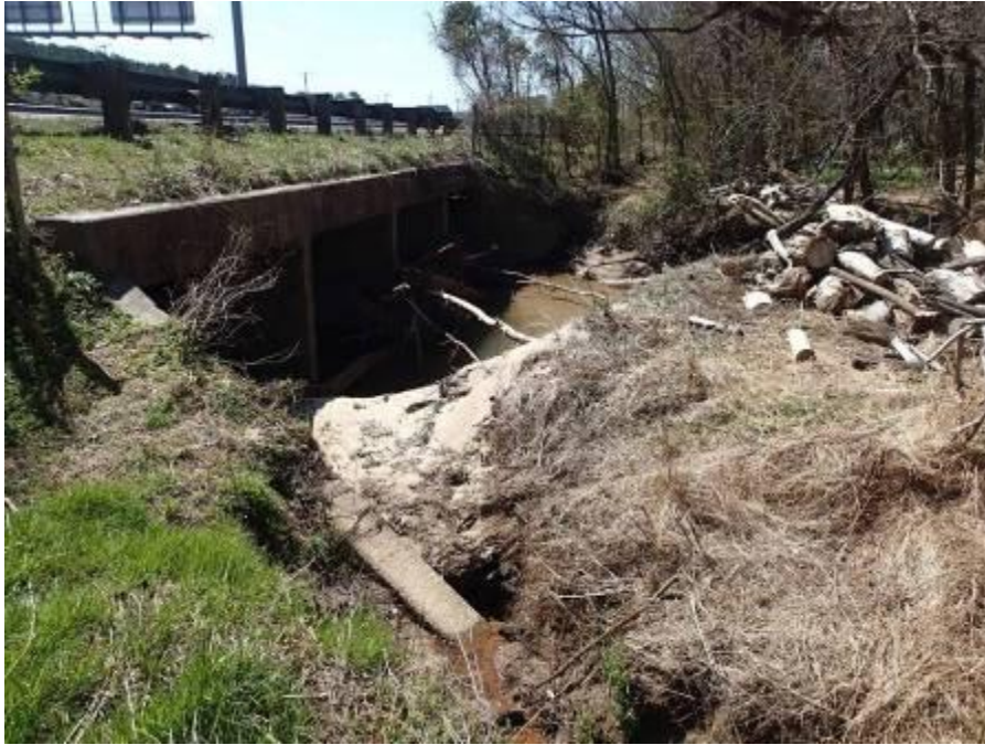
Station 0+00. View of 15-501 culvert from the left descending side.
