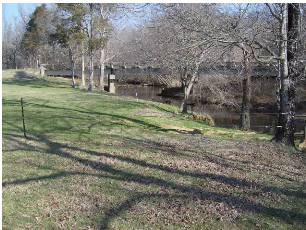
Facing west at the bridge over Sandy Creek. The easement intersects SR 2442 approximately 100 feet north of the structure.
