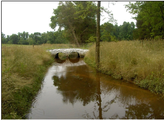
Cross Section #2 – Facing downstream
