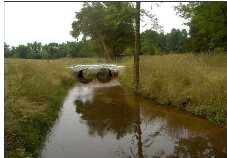
Cross Section 2 Facing Downstream
