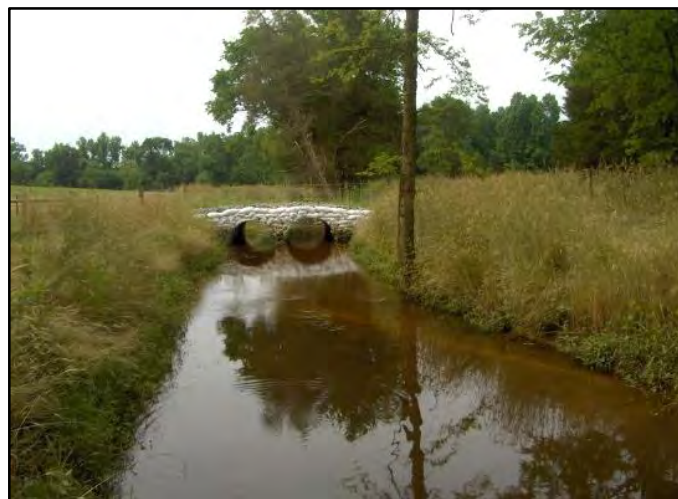
Cross Section 2 Facing Downstream
