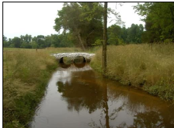
Cross Section 2 Facing Downstream
