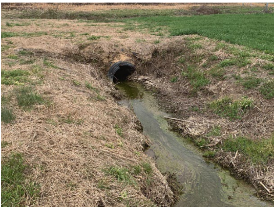
Culvert crossing at confluence of D4 and J1 March 17, 2022
