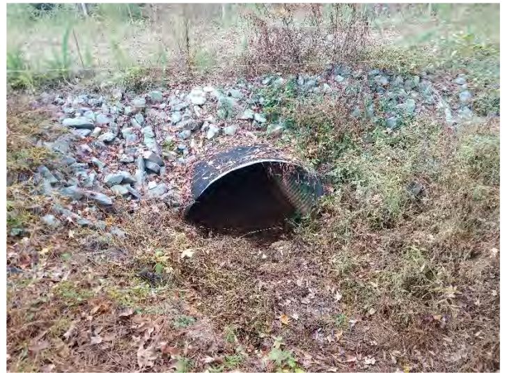
T5 Reach 3 – Looking Downstream (11/17/2021)
