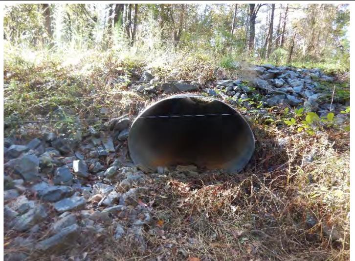
T4 Reach 3 – Looking Downstream (11/9/2021)
