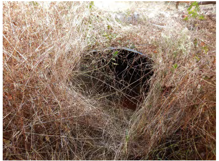
T6 Reach 2 – Looking Downstream (11/14/2023)
