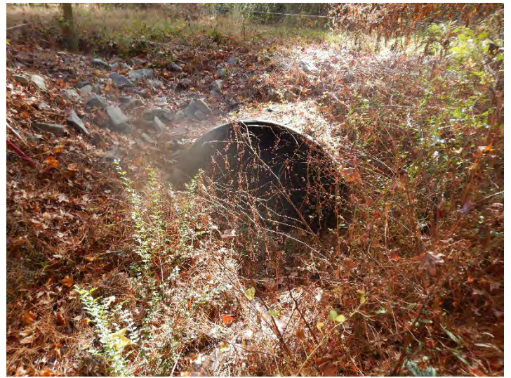
T5 Reach 3 – Looking Downstream (11/14/2023)
