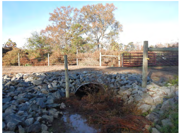
T1 Reach 1 – Looking Downstream (11/14/2023)
