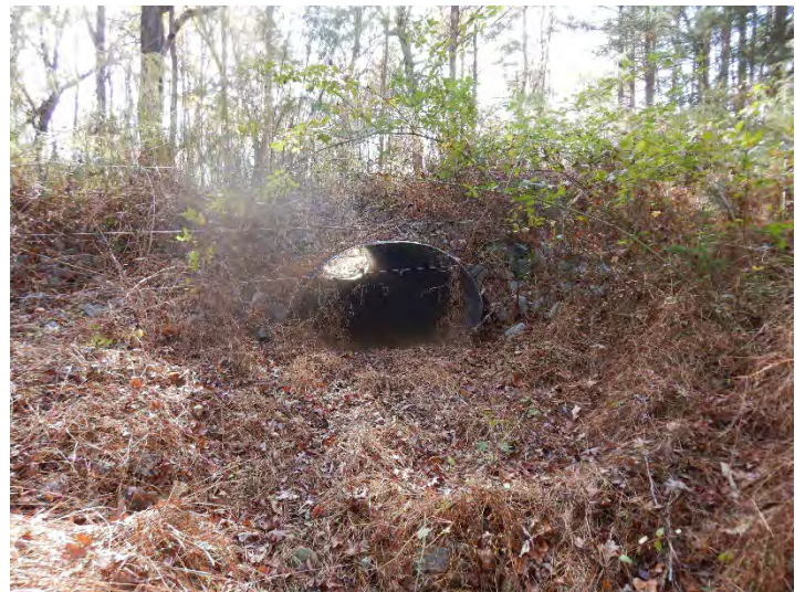
T4 Reach 3 – Looking Downstream (11/14/2023)
