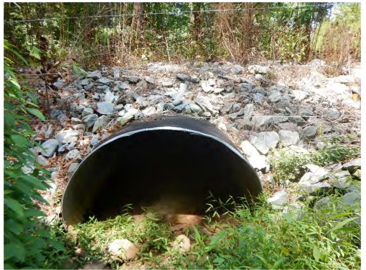
T5 Reach 3 – Looking Downstream (4/7/2022)
