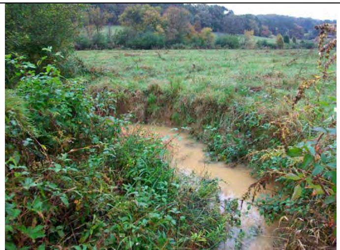
Photo 12-View of UT2 right bank erosion, facing downstream.
