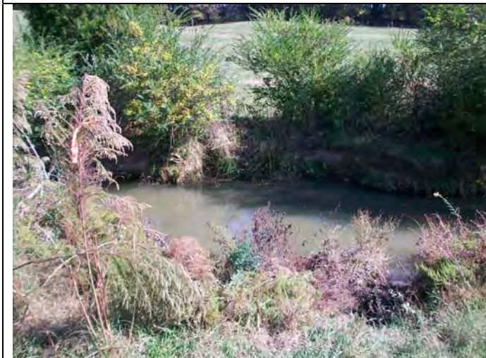
Photo 3-View of left bank erosion at Scaly Bark Creek XS 4.
