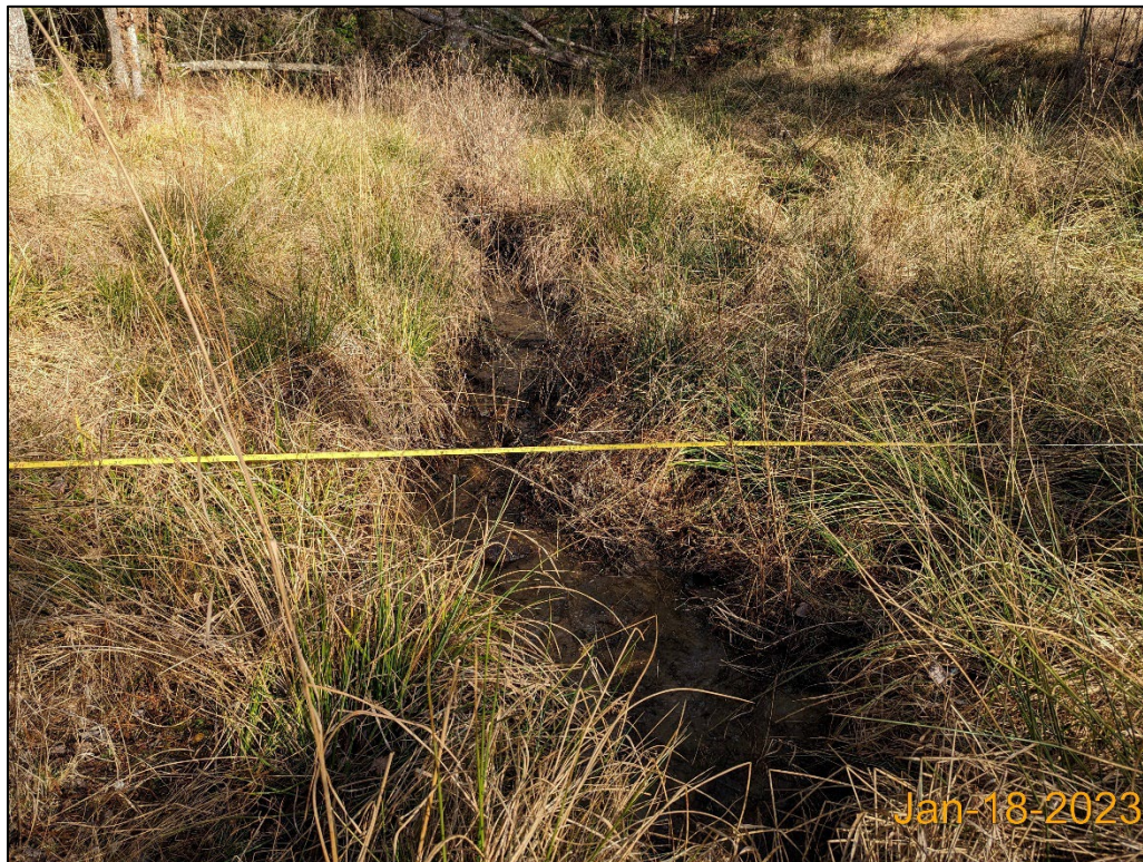
MY2 (2022) Lee Branch Station 300+25 facing upstream.
