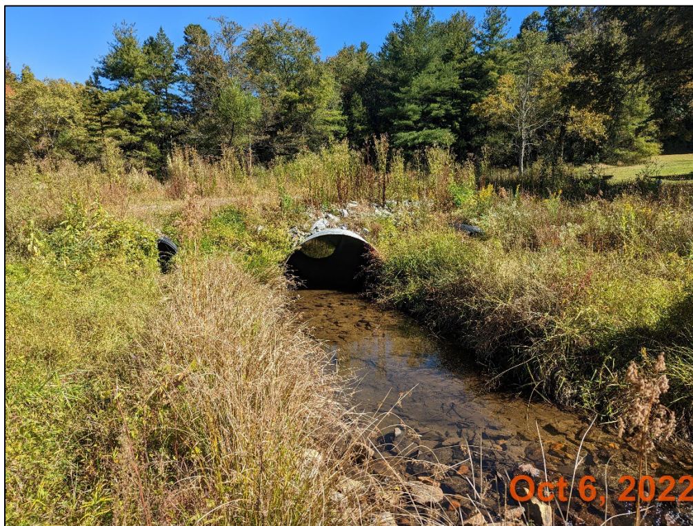
Photo Point 7.3 Facing upstream Sitton Branch culvert.
