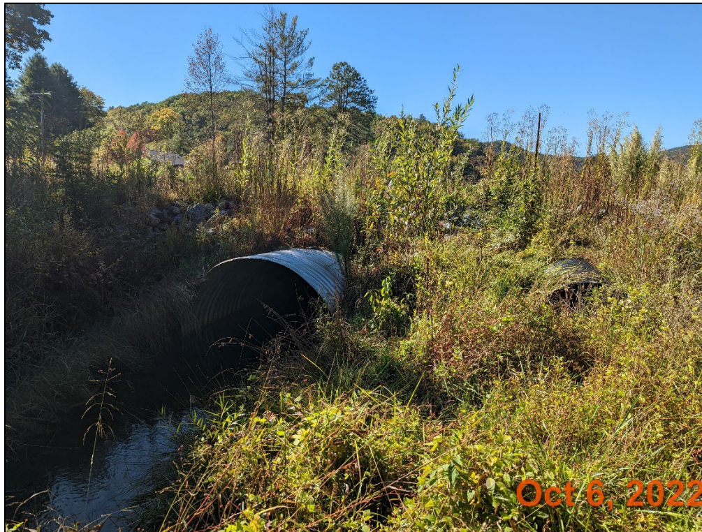
Photo Point 7.3 Facing downstream Sitton Branch culvert.
