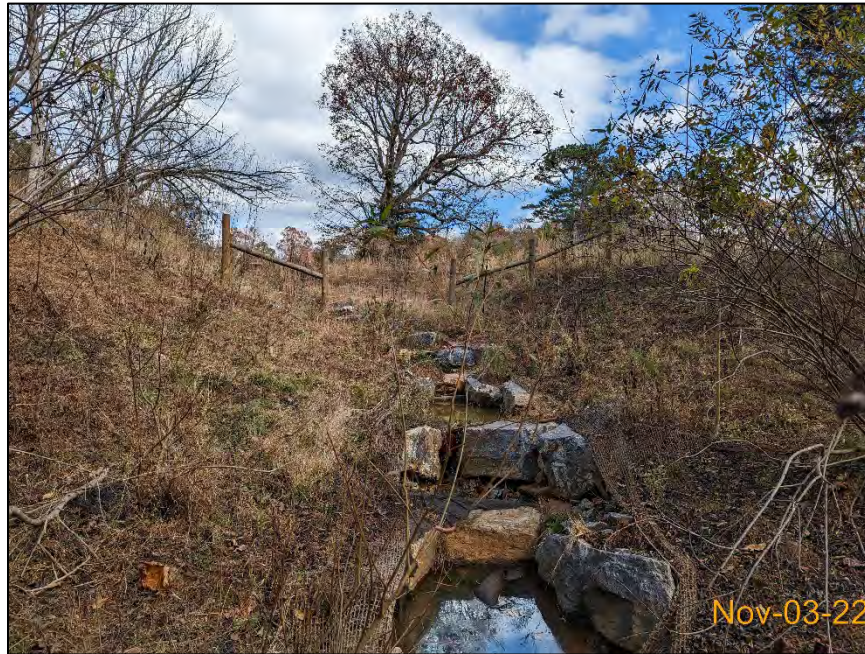
UT-10 – Permanent Photo Station 21 Supplemental Looking Upstream at head of project and 2021 Repair Area
