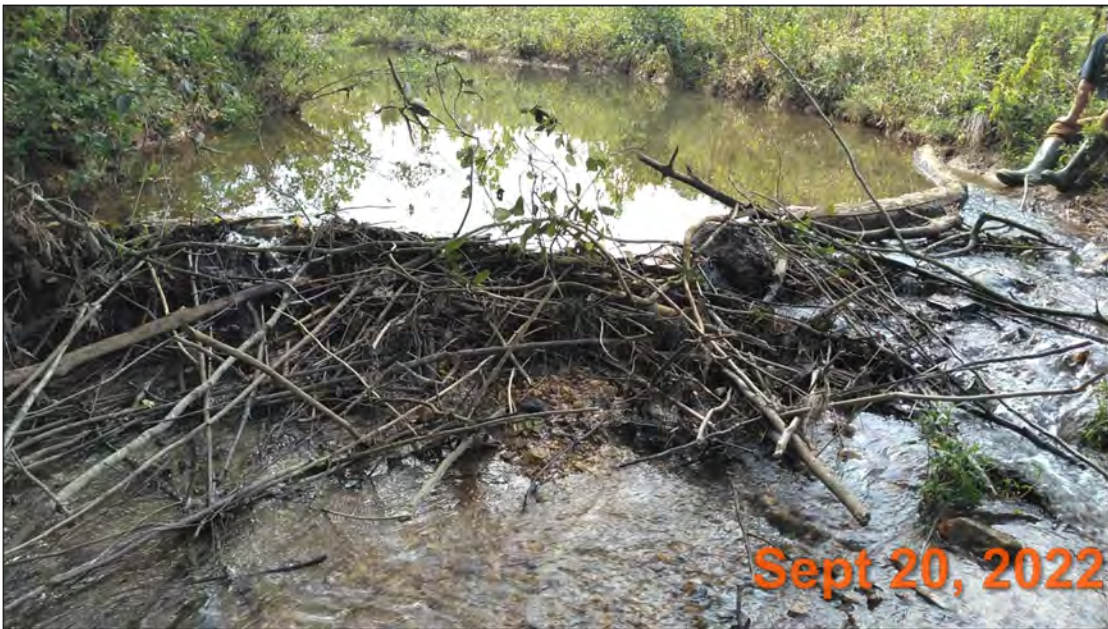
Shadrick Creek Reach 1 –Secondary beaver dam Station 36+50
