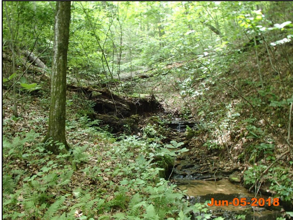
UT5 – Permanent Photo Station 30 Looking Upstream
