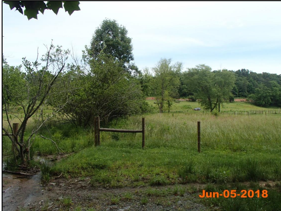
UT-7 – Permanent Photo Station 7 Looking Downstream from Crossing
