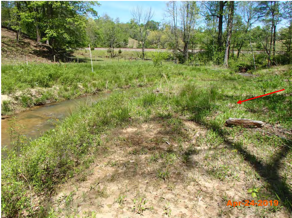
Photo #2 – Shadrick Creek Reach 1 STA 116+00 Wrack Lines
