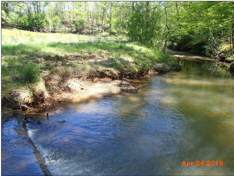
Shadrick Creek Reach 1 – Bank Erosion Station 39+00
