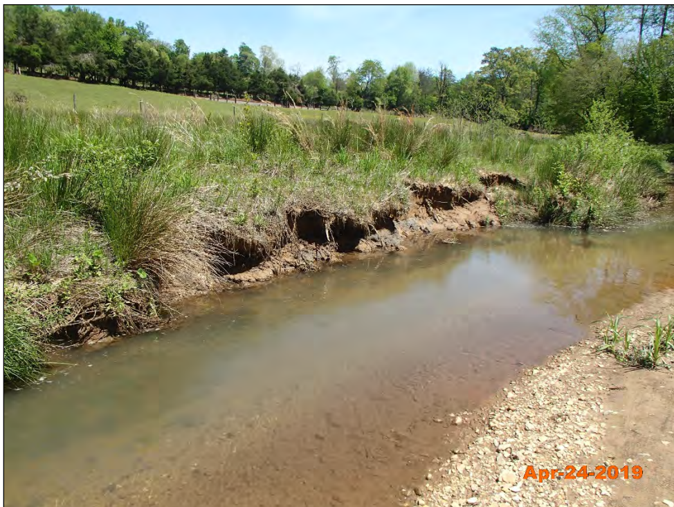
Shadrick Creek Reach 1 – Bank Erosion Station 33+75
