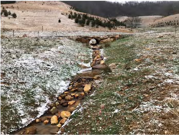
Photo Point 13 – UT4, view upstream (01/20/2020)
