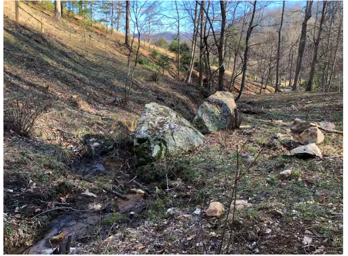
Photo Point 30 – UT5, view downstream (01/28/2020)
