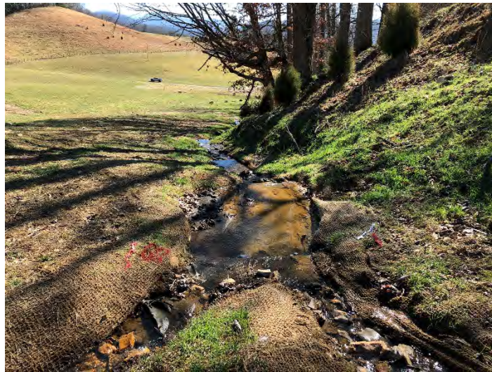
Photo Point 22 – SRB Reach 3, view downstream (01/28/2020)
