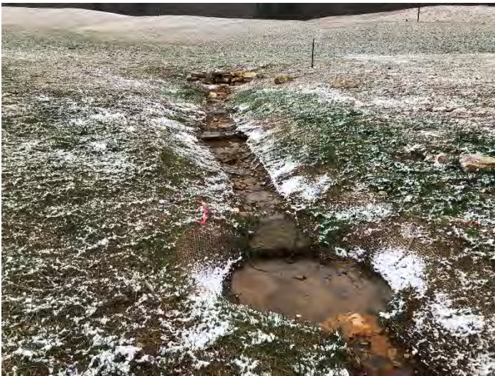
Photo Point 14 – UT8, view upstream (01/20/2020)
