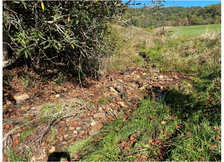
Shake Rag Reach 4 STA 923+75: Minor deposition at valley break
