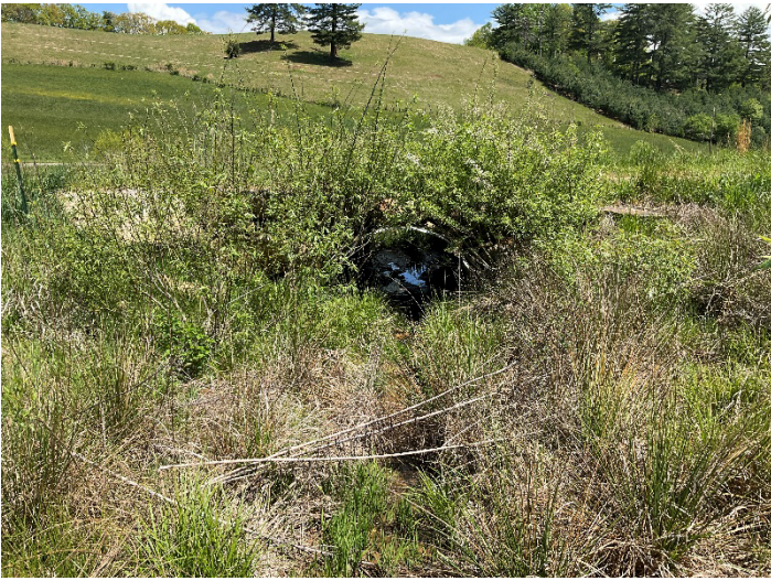
Culvert Crossing – UT4 at STA 407+75, inlet view (04/28/2023)
