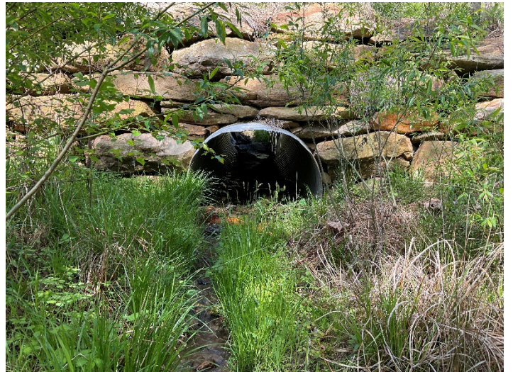
Culvert Crossing – UT2 Reach 2 at STA 204+15, outlet view (04/28/2023)
