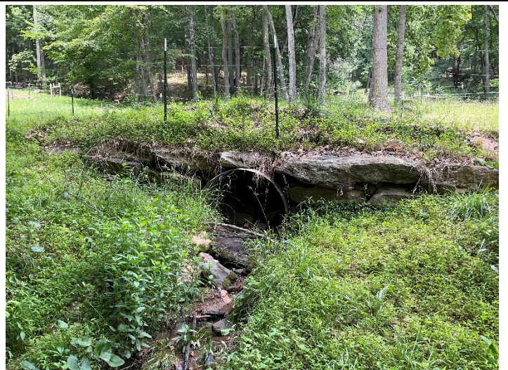
Culvert Crossing – UT6 at STA 605+75, outlet view (6/15/2023)
