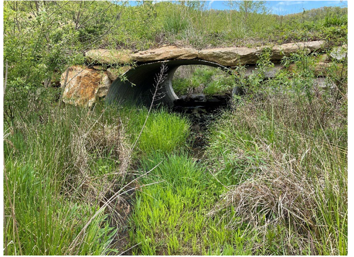
Culvert Crossing – SRB Reach 5 at STA 932+00, outlet view (04/28/2023)
