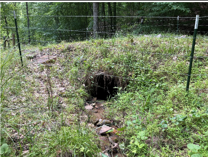
Culvert Crossing – UT6 at STA 605+75, inlet view (6/15/2023)
