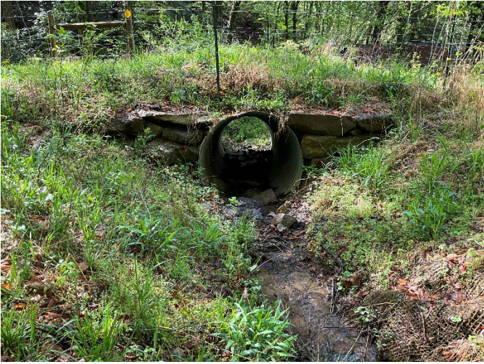
Culvert Crossing – UT1 Reach 1 at STA 106+75, inlet view (04/28/2023)
