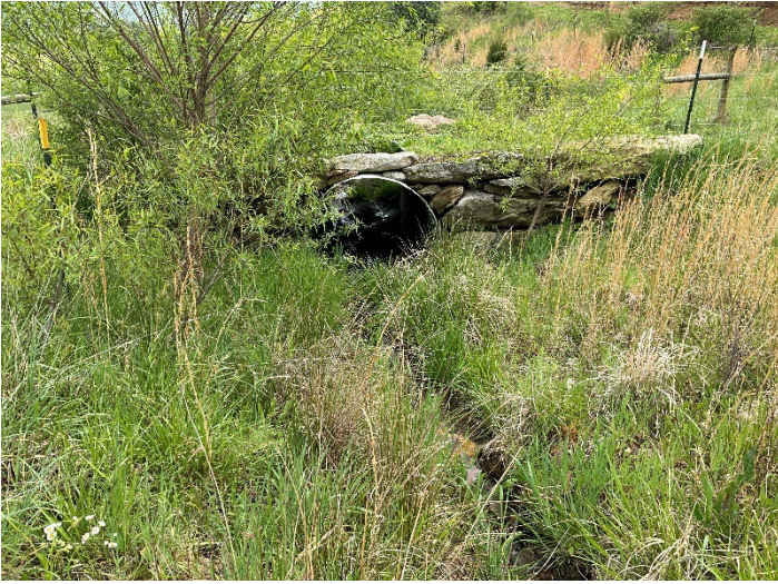
Culvert Crossing – SRB Reach 3 at STA 914+00, inlet view (04/28/2023)
