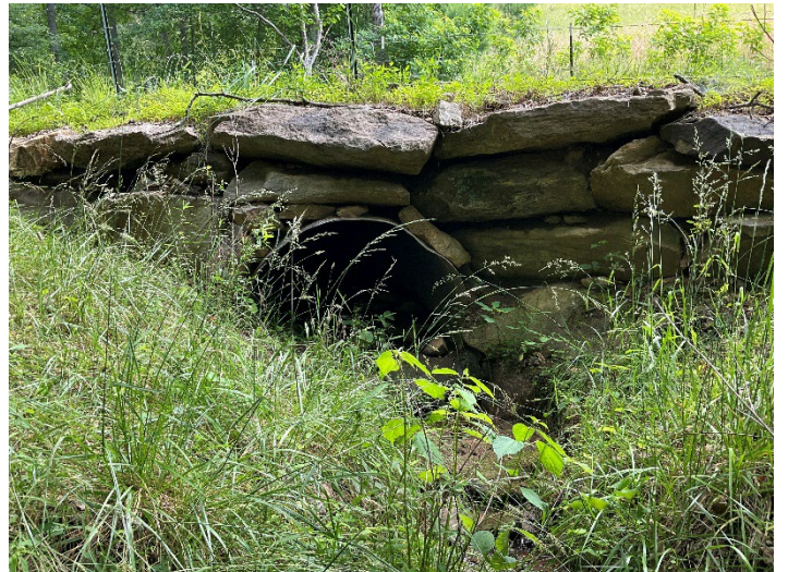
Culvert Crossing – UT5 at STA 504+00, outlet view (6/15/2023)
