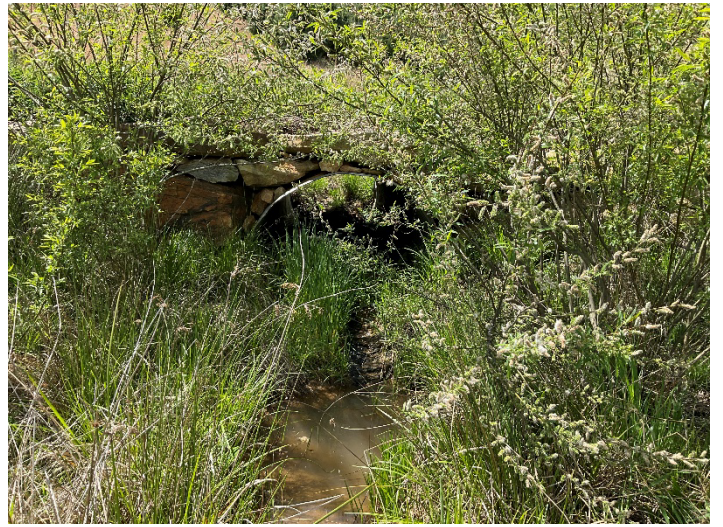
Culvert Crossing – UT4 at STA 407+75, outlet view (04/28/2023)
