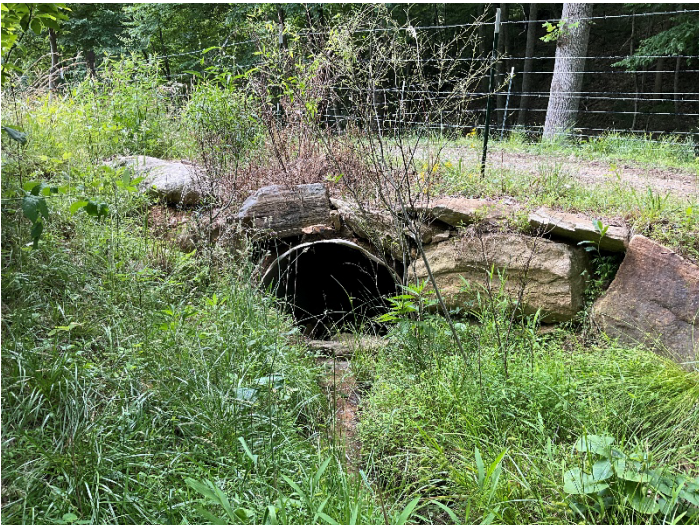
Culvert Crossing – UT5 at STA 504+00, inlet view (6/15/2023)
