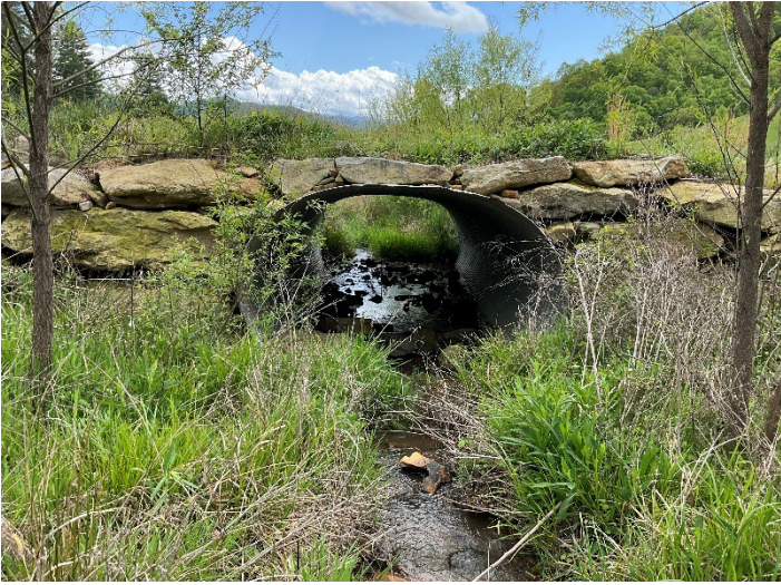
Culvert Crossing – SRB Reach 5 at STA 932+00, inlet view (04/28/2023)
