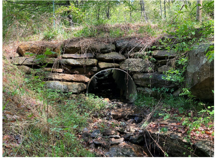
Culvert Crossing – UT1 Reach 1 at STA 106+75, outlet view (04/28/2023)
