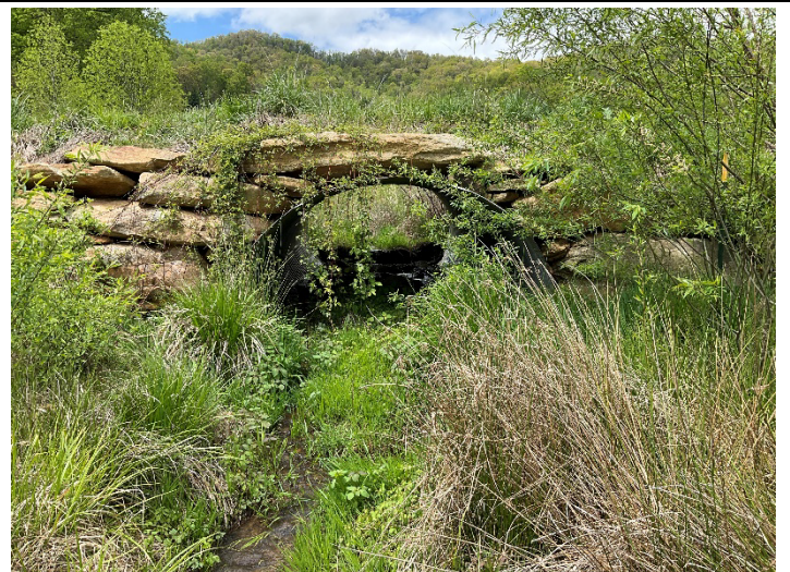
Culvert Crossing – SRB Reach 5 at STA 928+25, outlet view (04/28/2023)
