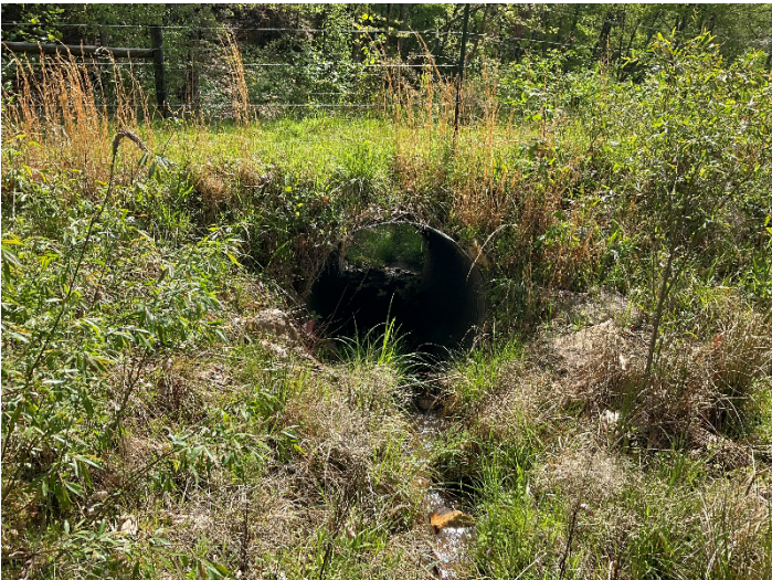
Culvert Crossing – UT2 Reach 2 at STA 204+15, inlet view (04/28/2023)
