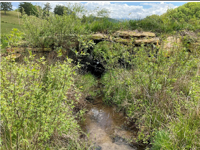
Culvert Crossing – SRB Reach 5 at STA 928+25, inlet view (04/28/2023)
