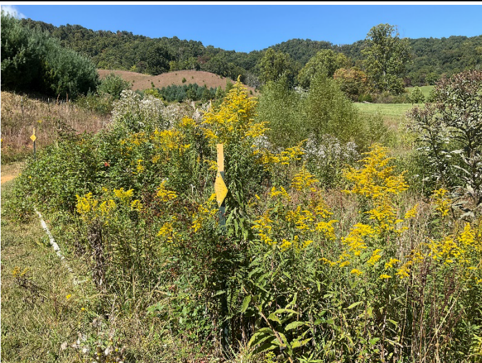
Pipe removed from easement – UT4, view up-valley (10/02/2023)
