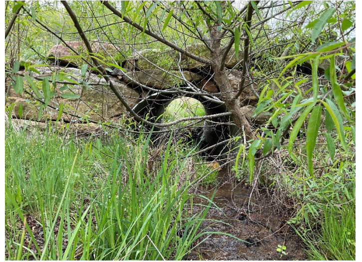
Culvert Crossing – SRB Reach 3 at STA 914+00, outlet view (04/28/2023)
