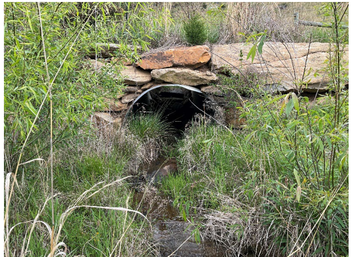
Culvert Crossing – UT3 Reach 2 at STA 309+25, outlet view (04/28/2023)
