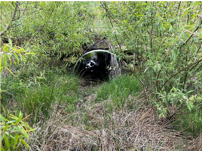
Culvert Crossing – UT3 Reach 2 at STA 309+25, inlet view (04/28/2023)
