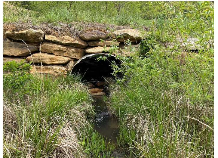
Culvert Crossing – SRB Reach 3 at STA 920+25, outlet view (04/28/2023)
