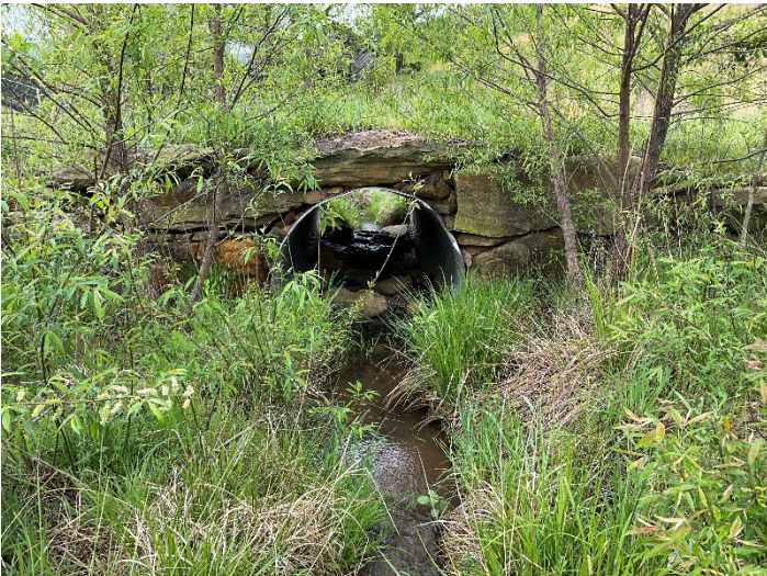
Culvert Crossing – SRB Reach 3 at STA 920+25, inlet view (04/28/2023)
