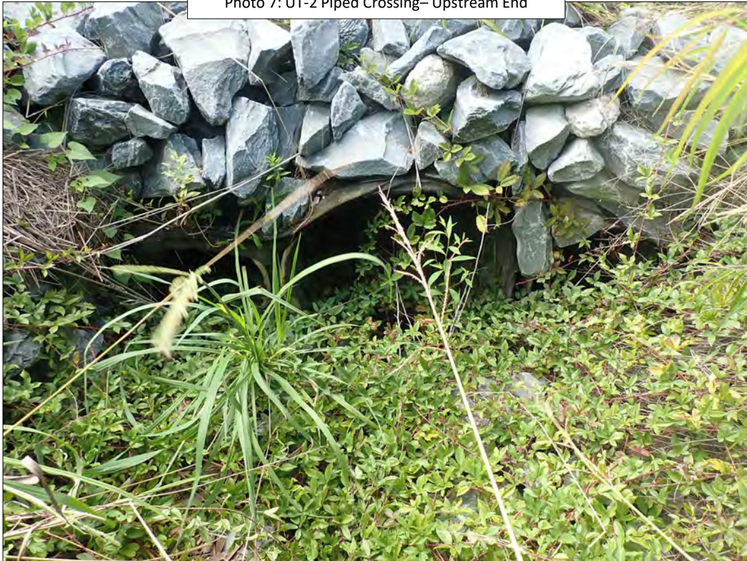
Photo 7: UT-2 Piped Crossing– Upstream End
