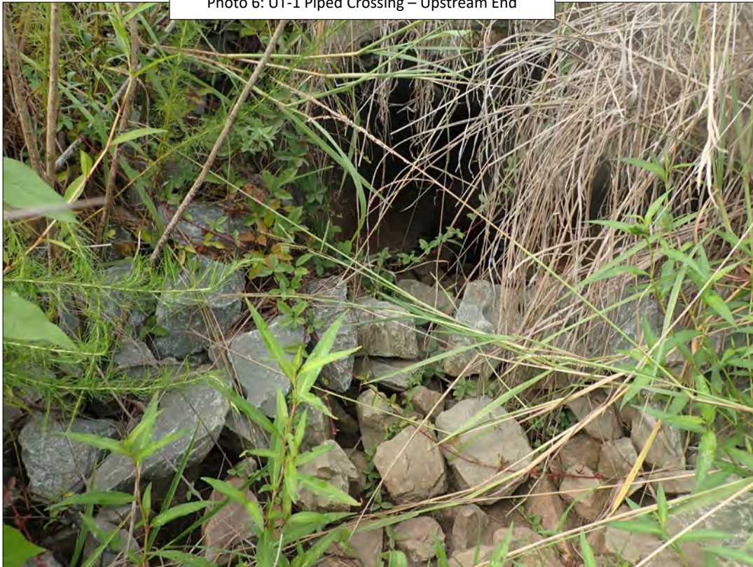
Photo 6: UT-1 Piped Crossing – Upstream End
