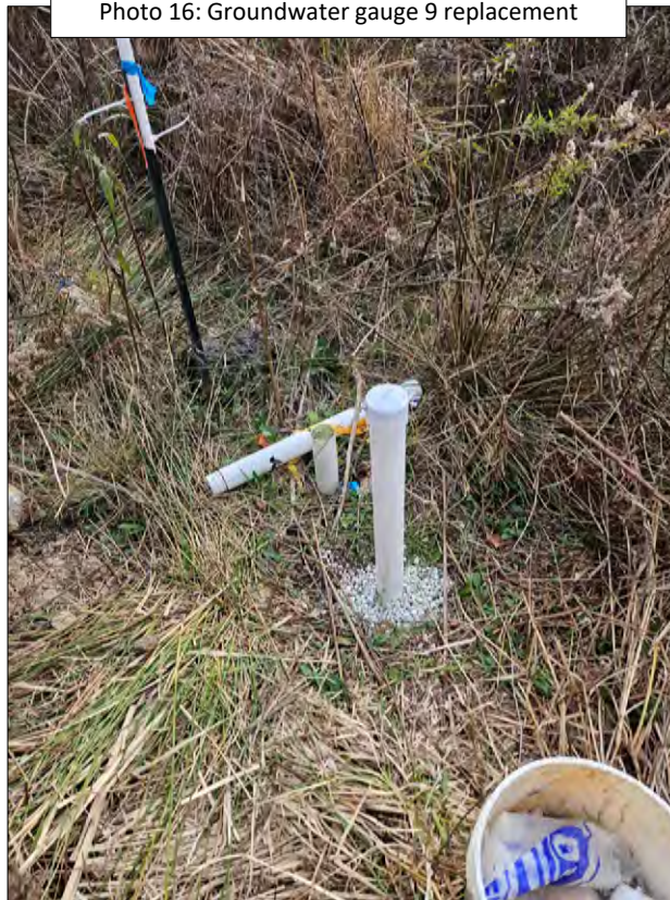
Photo 16: Groundwater gauge 9 replacement
