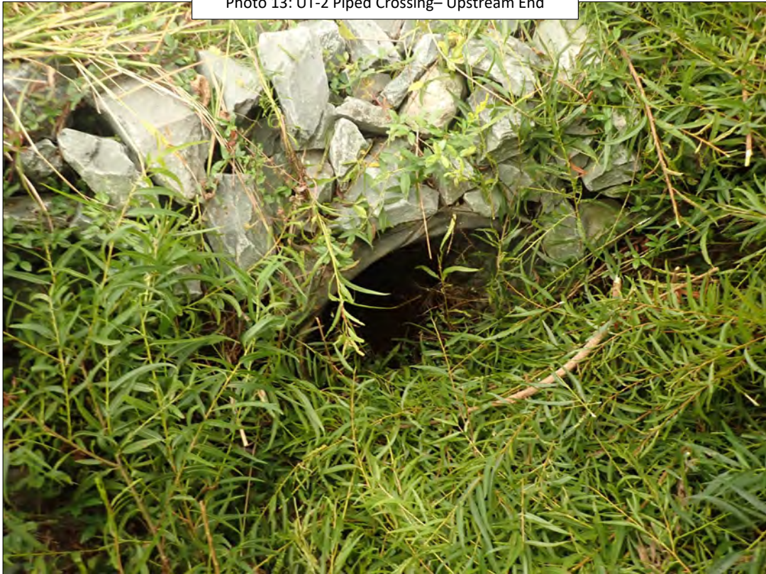
Photo 13: UT-2 Piped Crossing– Upstream End
